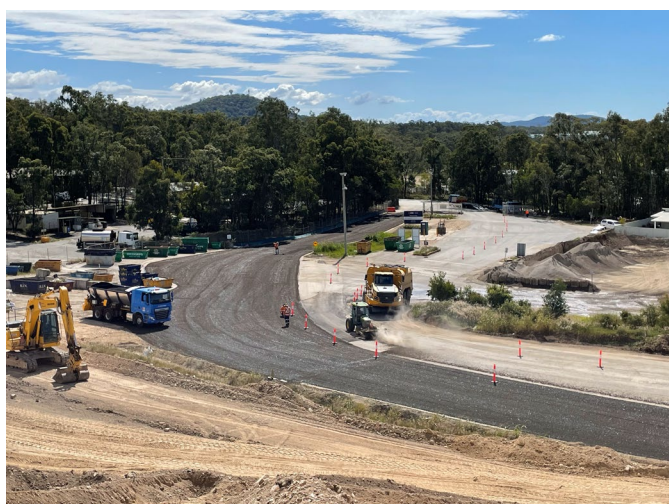
Figure 3 - Two coat bitumen seal between weighbridge and exist and on weighbridge slip lane
