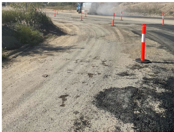
Figure 2 - Hot mix pothole repairs on road from wheel wash to exit
