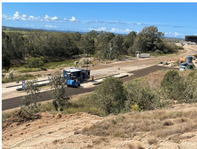
Figure 1 - Hot mix bitumen seal between wheel wash and weighbridge
