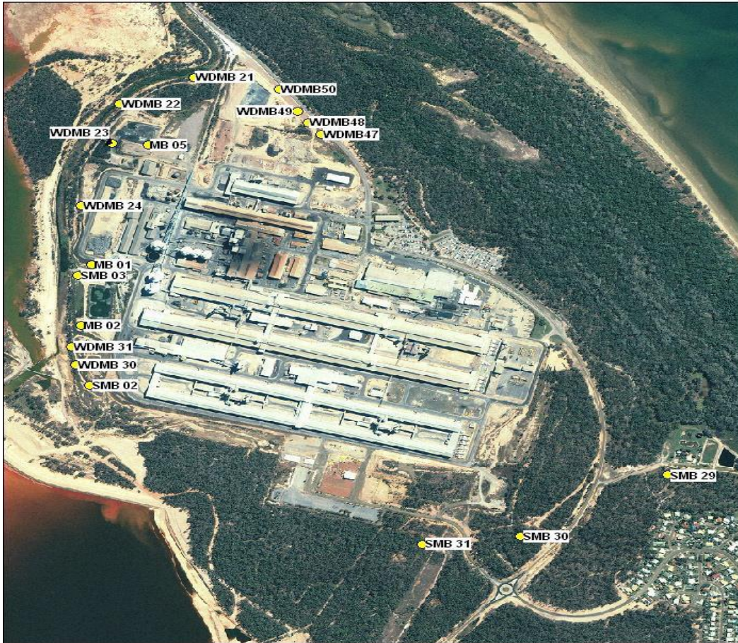
BSL License Groundwater Monitoring Bores
