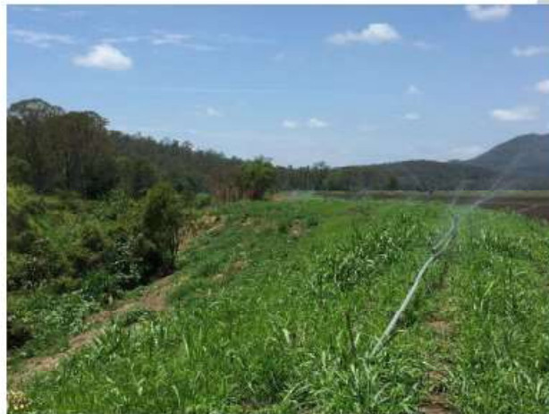
Figure 11: An example of a battered bank on Laidley Creek
