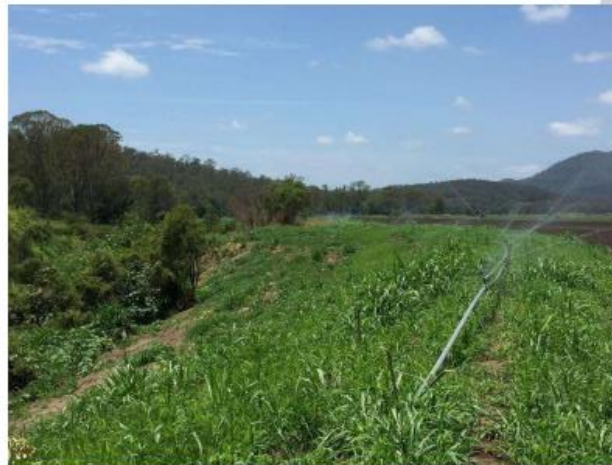
Figure 11: An example of a battered bank on Laidley Creek
