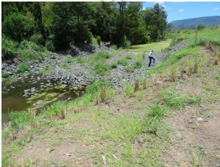
Figure 15: An example of a grade control structure constructed upstream in Laidley creek in 2013
