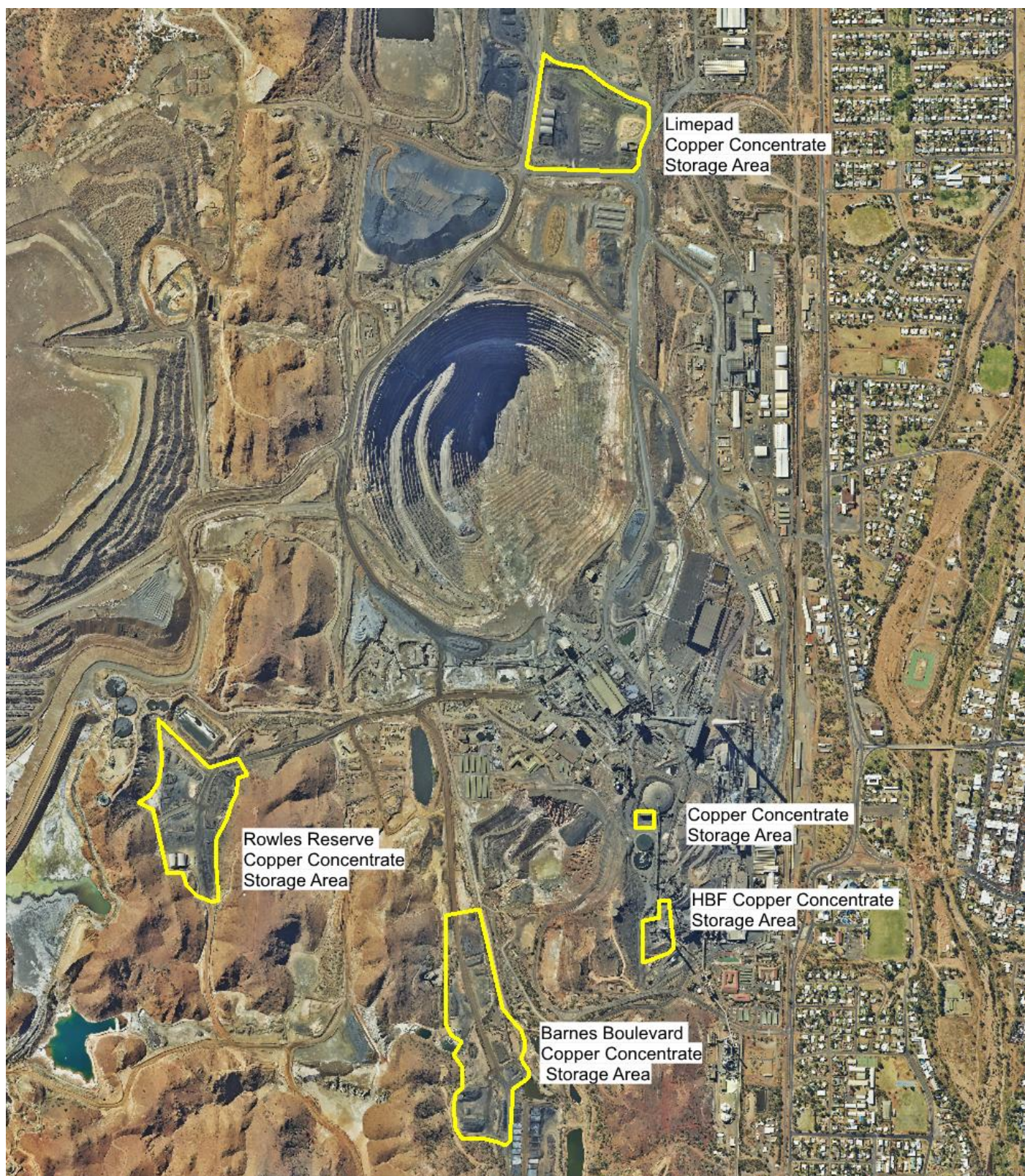
Schedule K – Figure 8 (Designated Copper Storage Areas)
