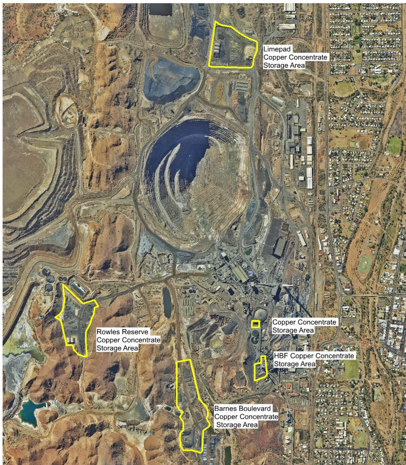
Schedule K – Figure 8 (Designated Copper Storage Areas)
