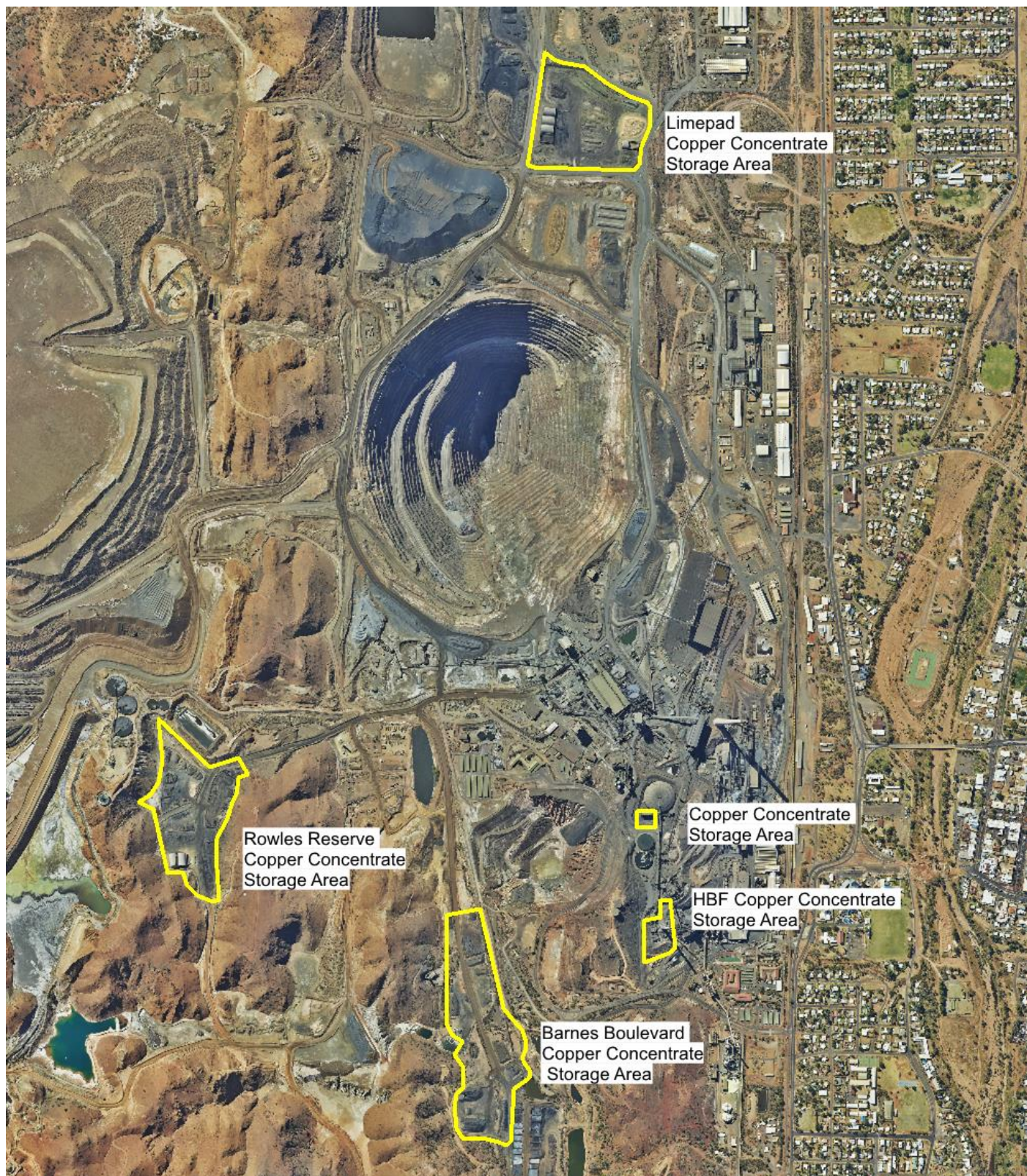
Schedule K – Figure 8 (Designated Copper Storage Areas)
