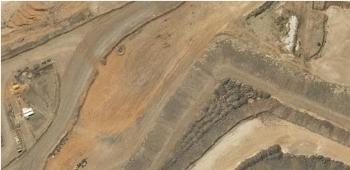
Map 7: Contractor demountable toilet block- irrigation area.
