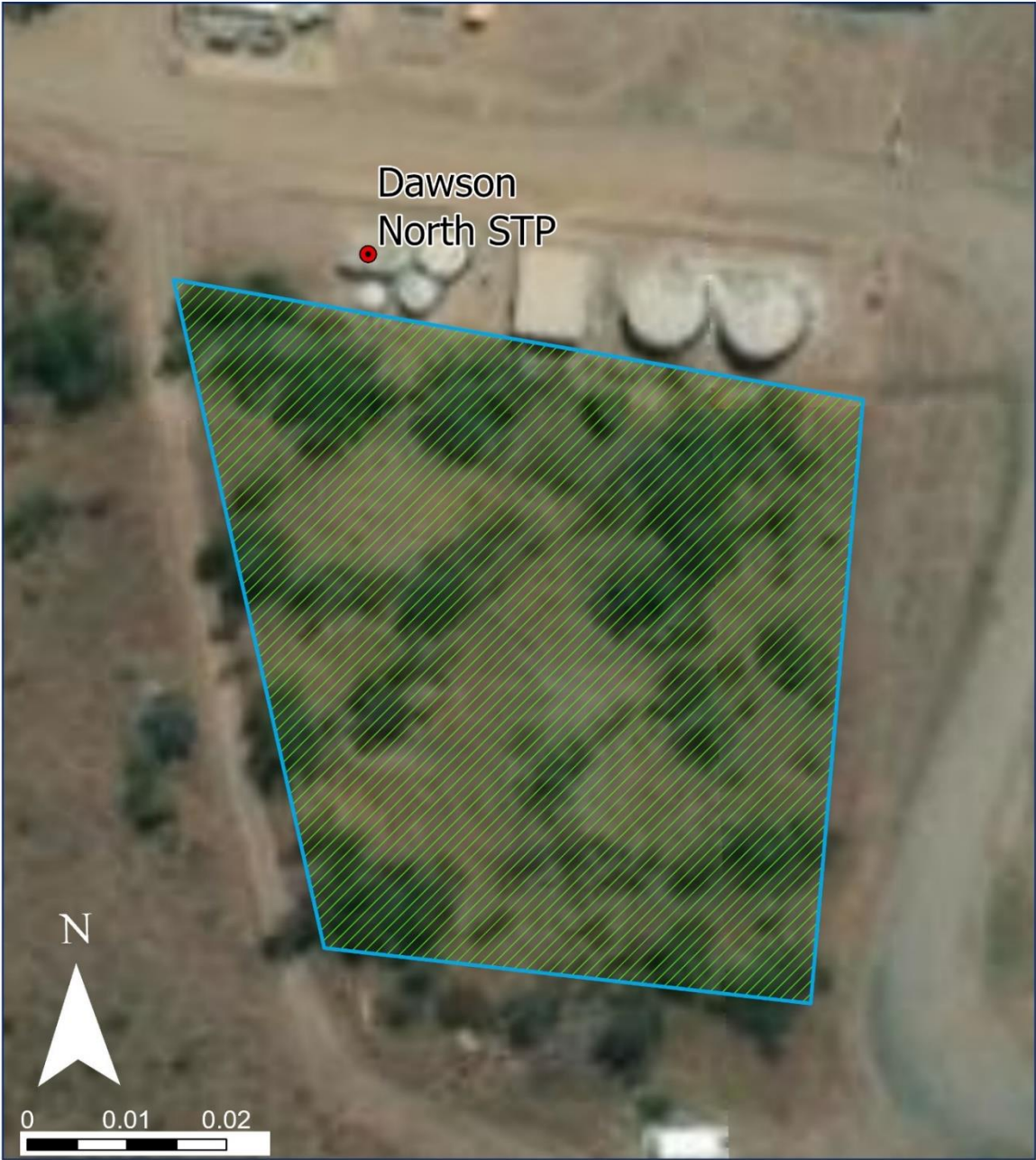
Figure 3b Dawson North STP
