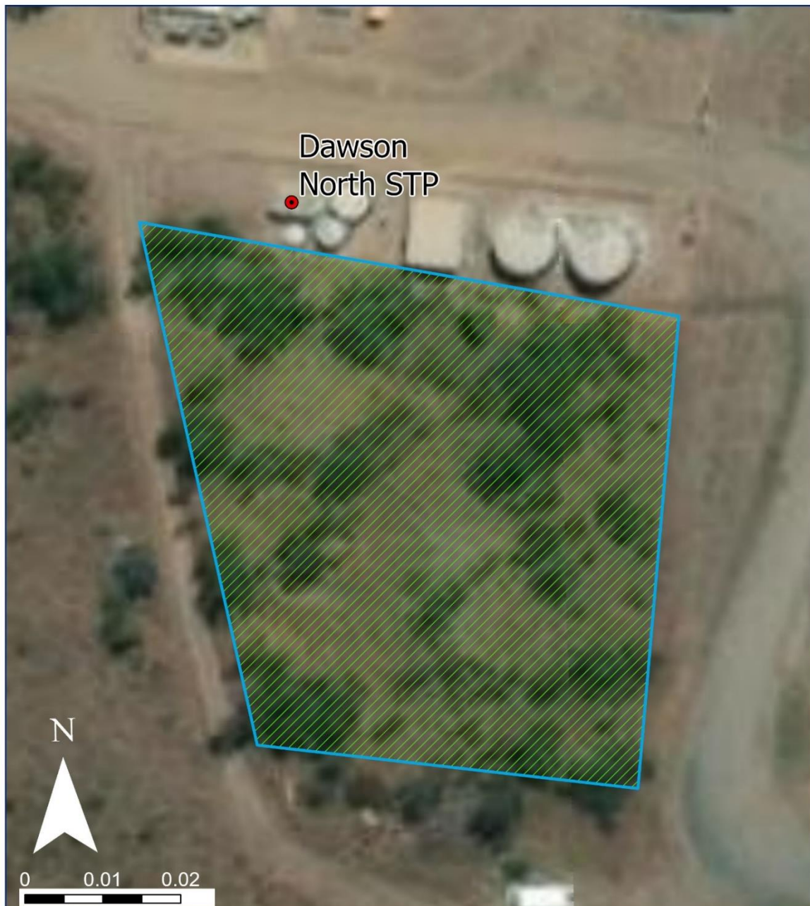
Figure 3b Dawson North STP
