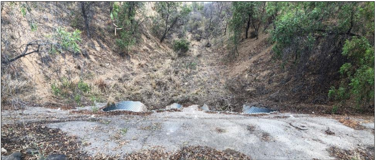
Figure 11-11 - Downstream (south) side of access road culvert with twin CMPs and lower side slope protected by shotcrete cover
