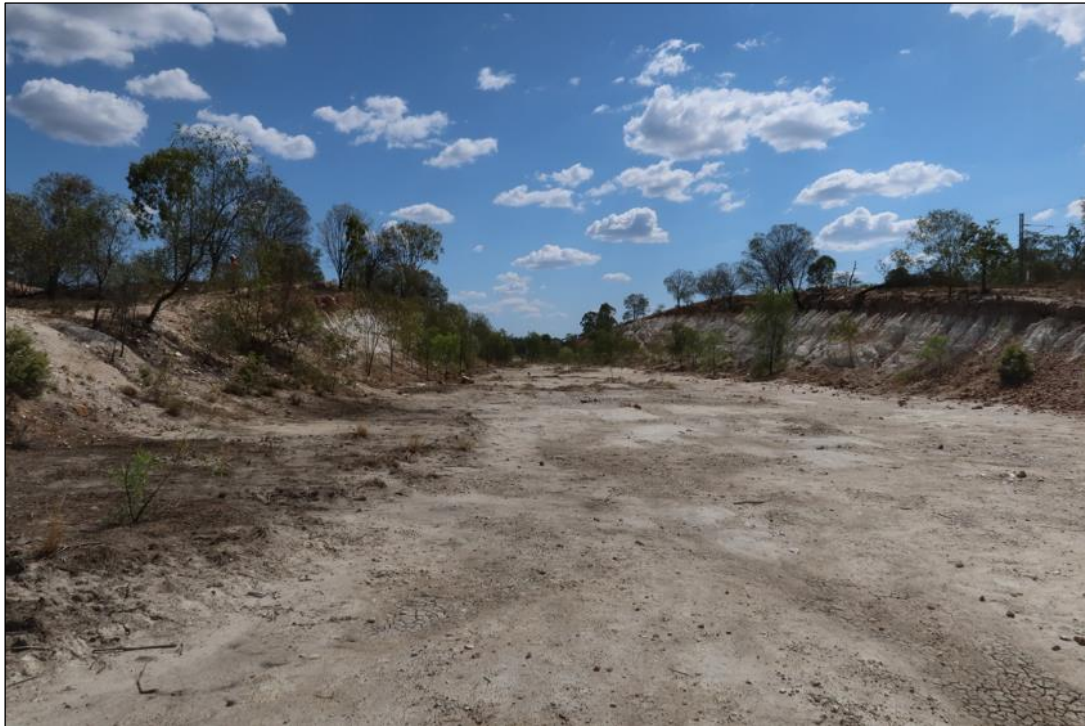
Figure 11-4 - East part of northwest channel cut viewed towards west showing batter and floor condition in weathered coal measures rocks
