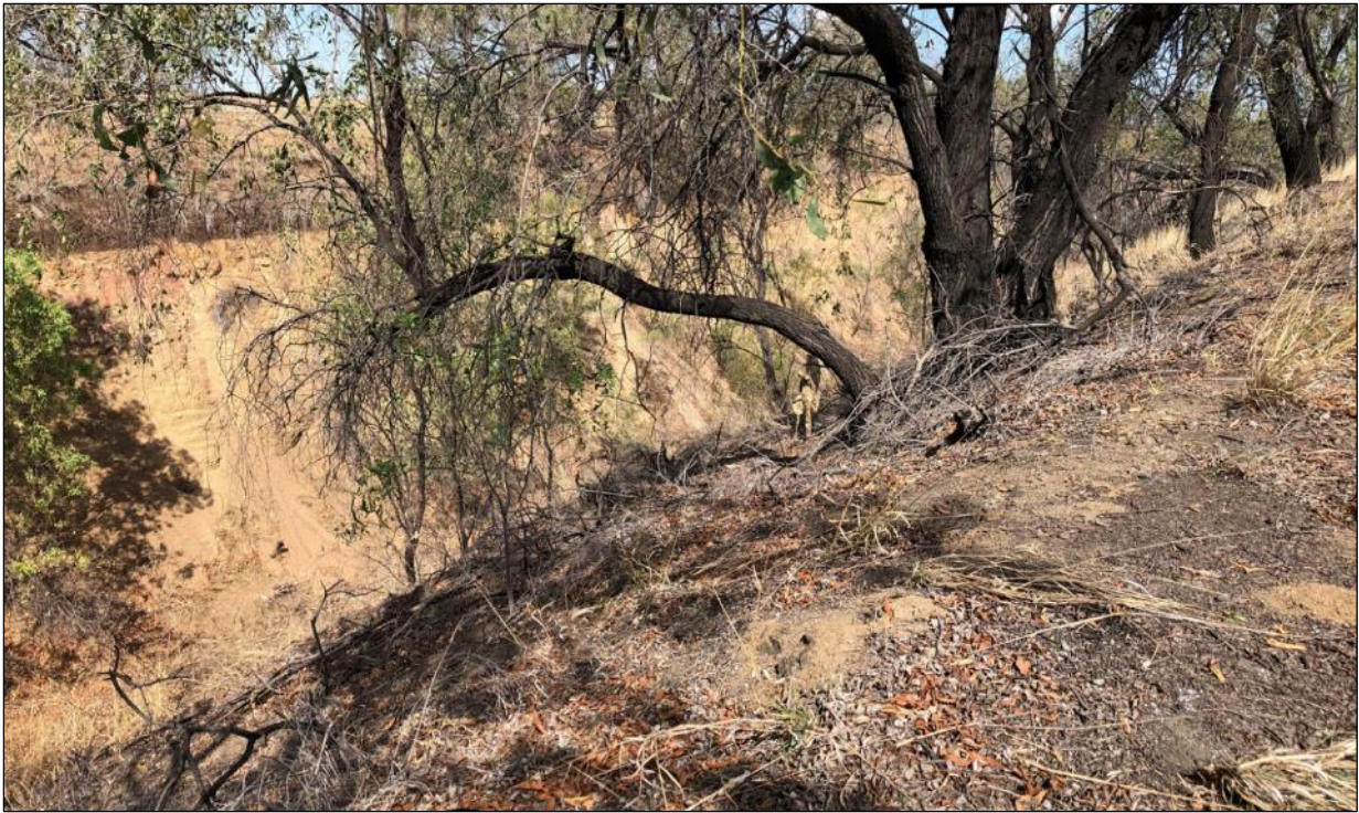
Figure 11-8 - Southeast channel cut in weathered basalt with nominal 2v:1h batters (view downstream towards southeast)
