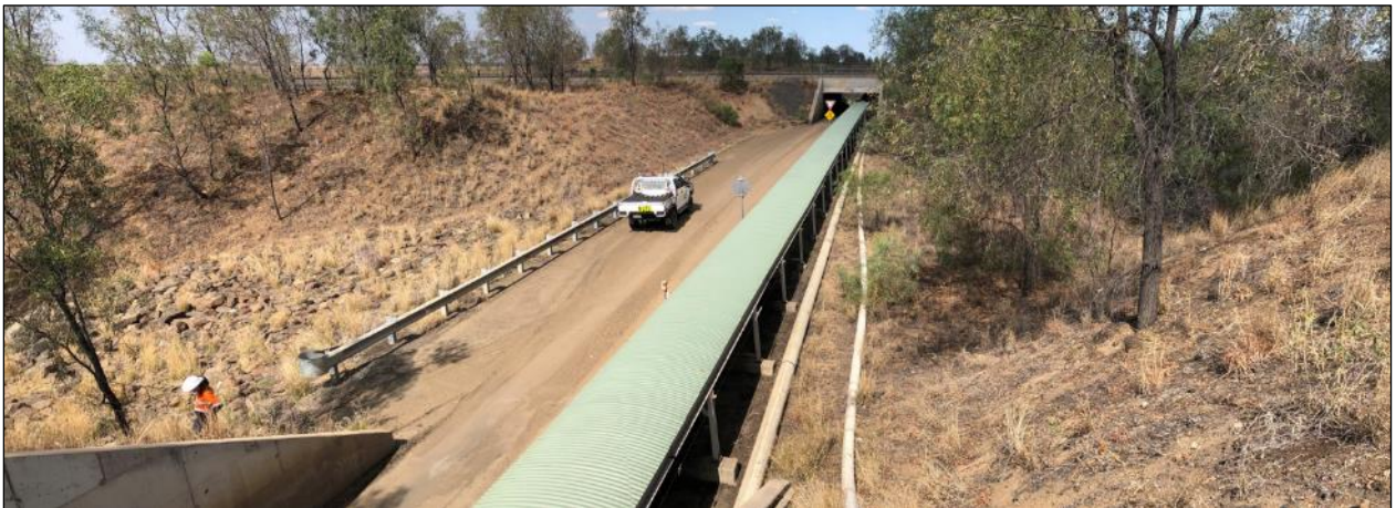
Figure 11-9 - Culvert crossing of southeast channel cut by overland conveyor (OLC) and access road, with upper side slopes protected by basalt rock fill
