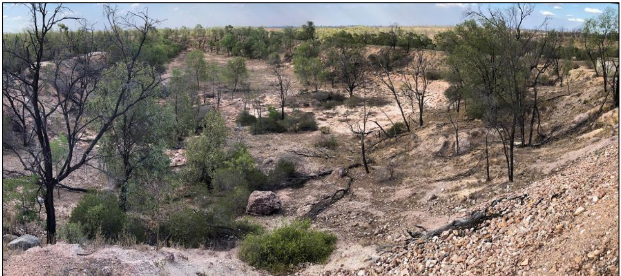
Figure 10-7 - Cement Hill eastern tailings cell viewed towards north showing northeast perimeter exclusion bund
