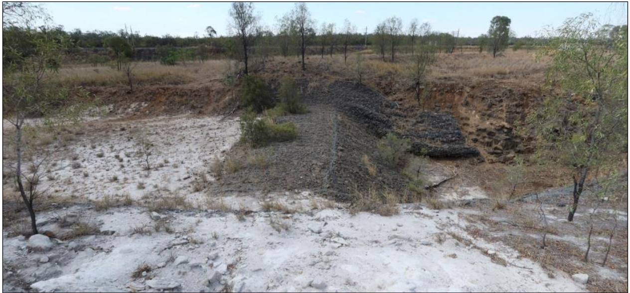
Figure 11-6 - Gabion and reno mattress drop structure at transition from merge zone into southeast channel cut and transition from sandstone to basalt materials
