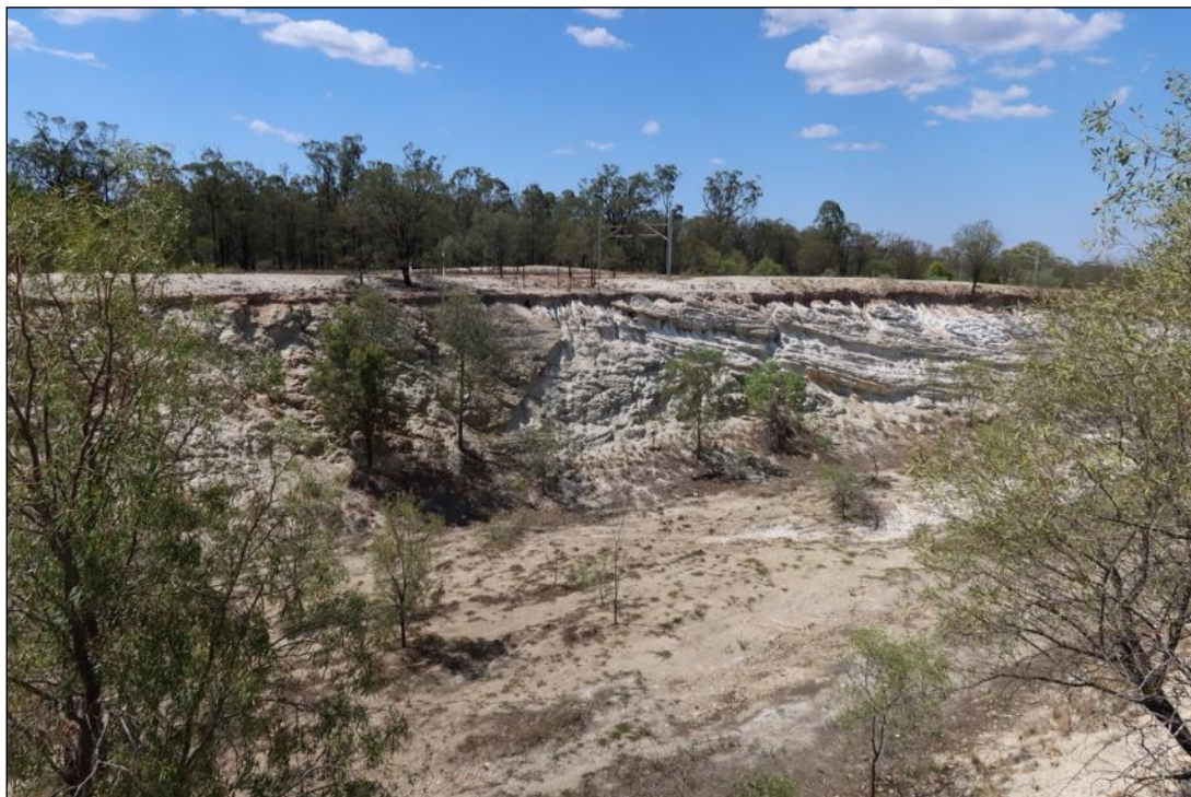
Figure 11-3 - Central part of northwest channel cut viewed towards northeast showing faulted transition from Anakie Metamorphics to Blair Athol coal measures rocks and erosion of batters
