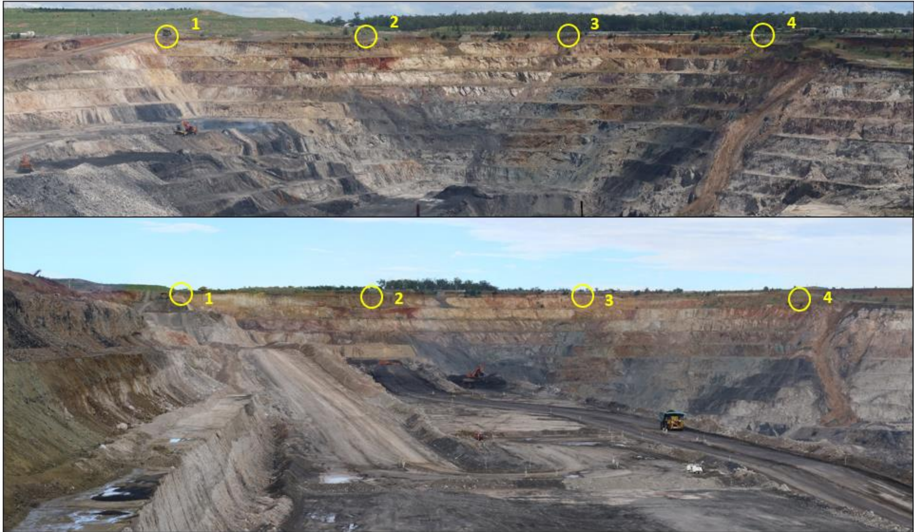
Figure 8-1 - West Wall March 2021 marked-up locations of weathered Anakie Metamorphics recommended for 1v:3h cutback treatment
