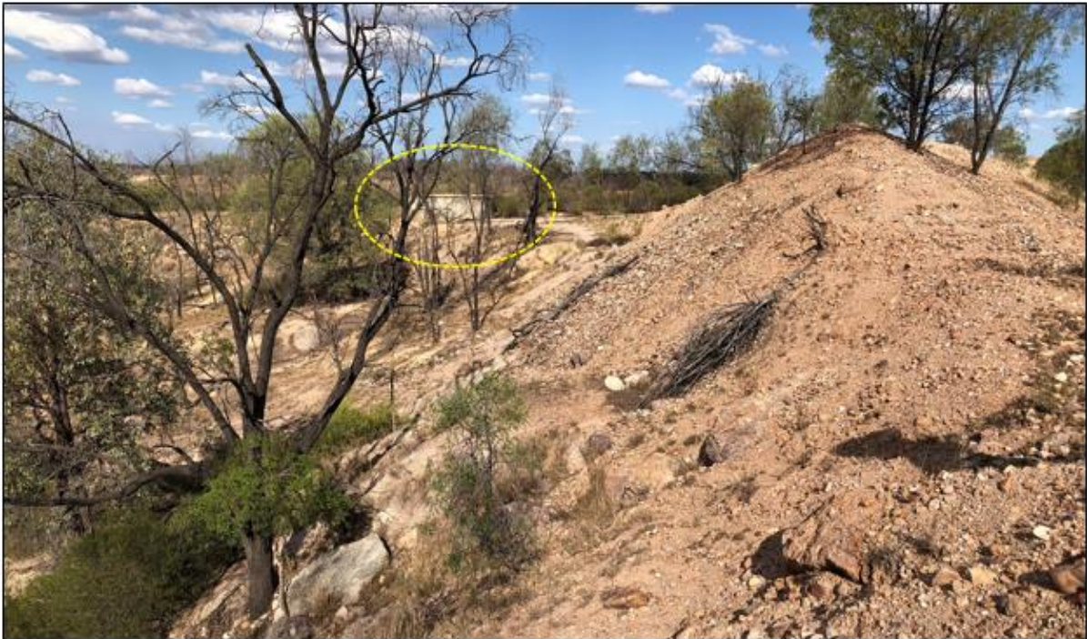
Figure 10-8 - Cement Hill dumped waste overlying southeast containment wall of tailings cell and remnant concrete tank (circled)
