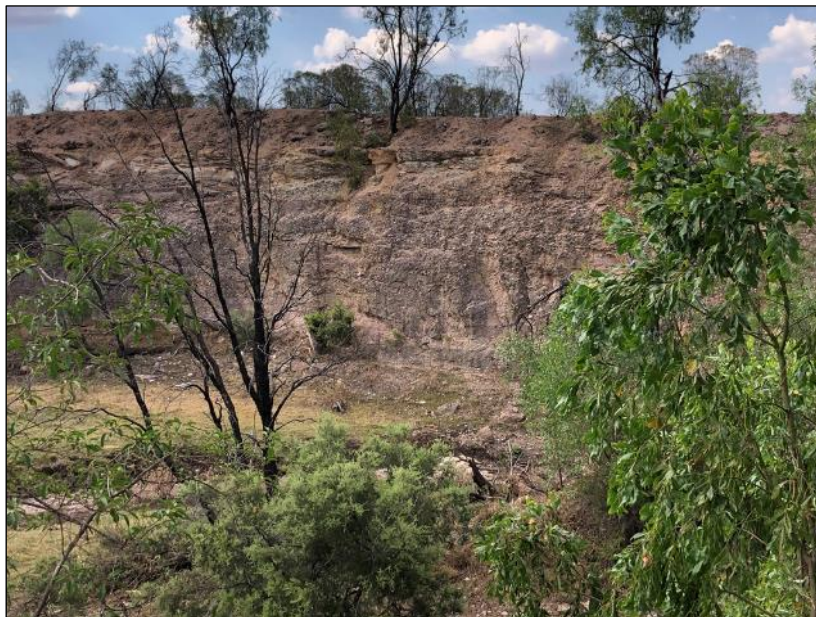
Figure 10-5 - Cement Hill "ramp" at west void margin provides flow path for flood overflow into void from tributary creek
