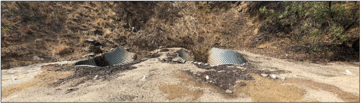
Figure 11-10 - Upstream (north) side of access road culvert with twin CMPs and lower side slope protected by shotcrete cover
