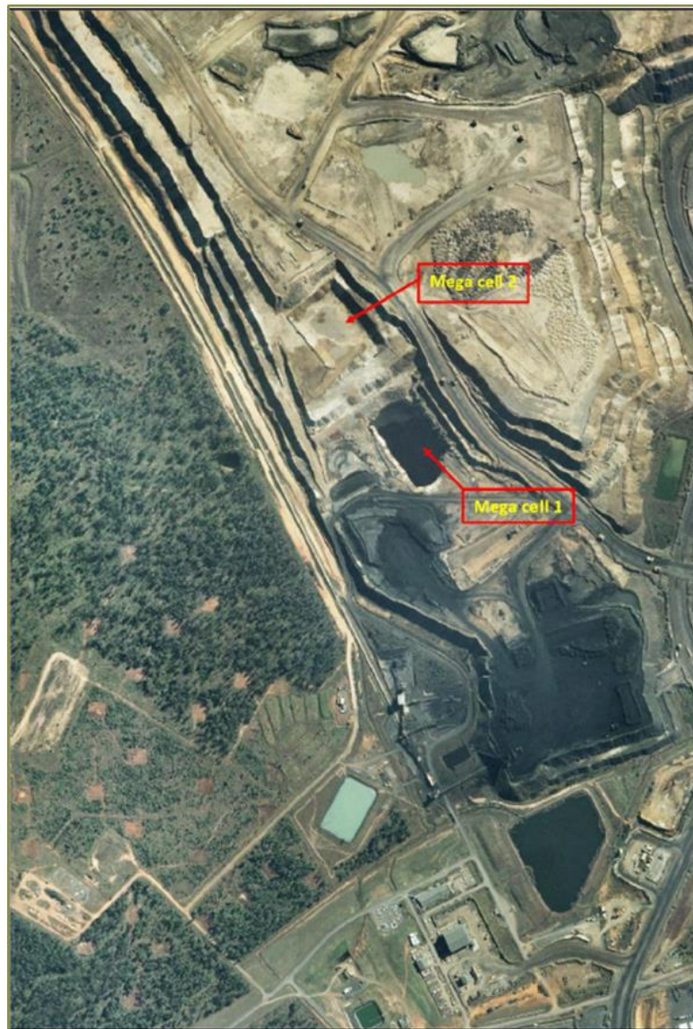
Figure 2-2 – Megacell 1 at completion and prior to encapsulation (circa 2013)
