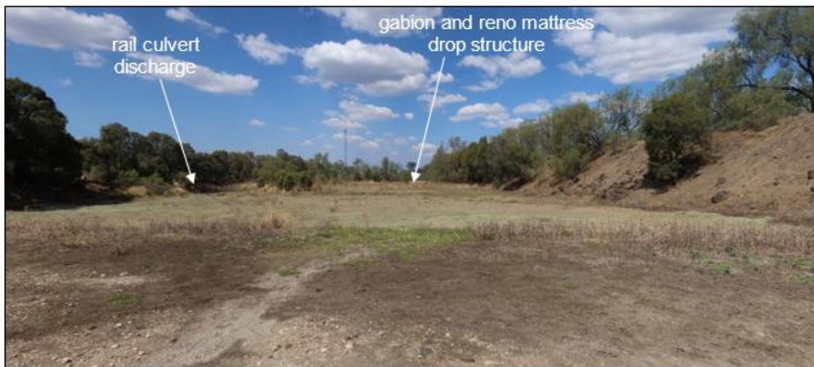
Figure 11-5 - Northwest channel cut merge zone with north tributary and transition to flatter batter in weathered basalt on south (right) bank
