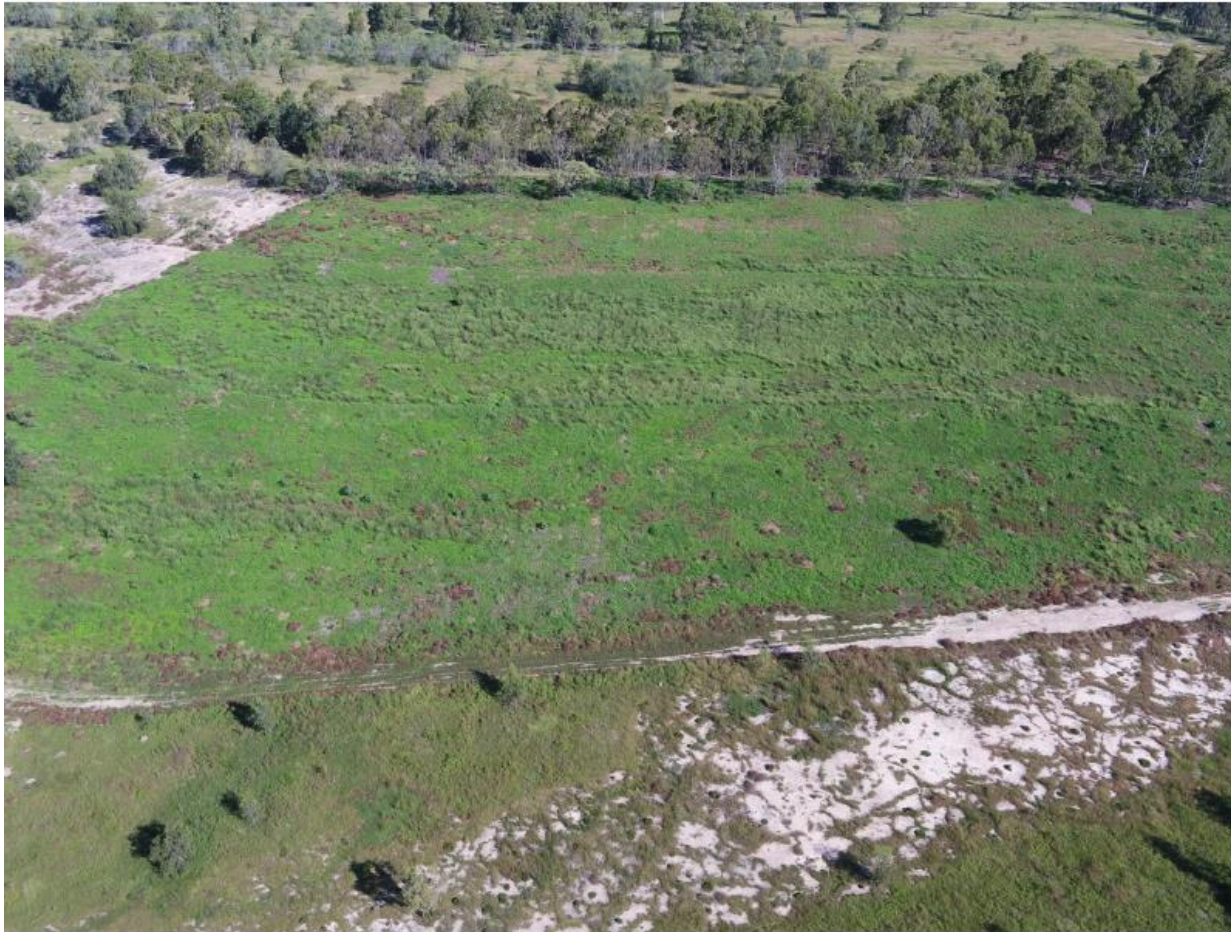
APPENDIX 2 - IMAGE 8: RECENTLY REPAIRED OPD NORTHERN BATTER SLOPE
