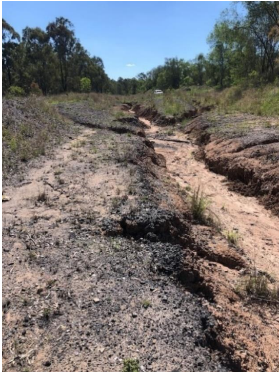
APPENDIX 2 - IMAGE 25: SOUTHERN DRAIN IN IBSD AREA BEFORE REHABILITATION, NOVEMBER 2018
