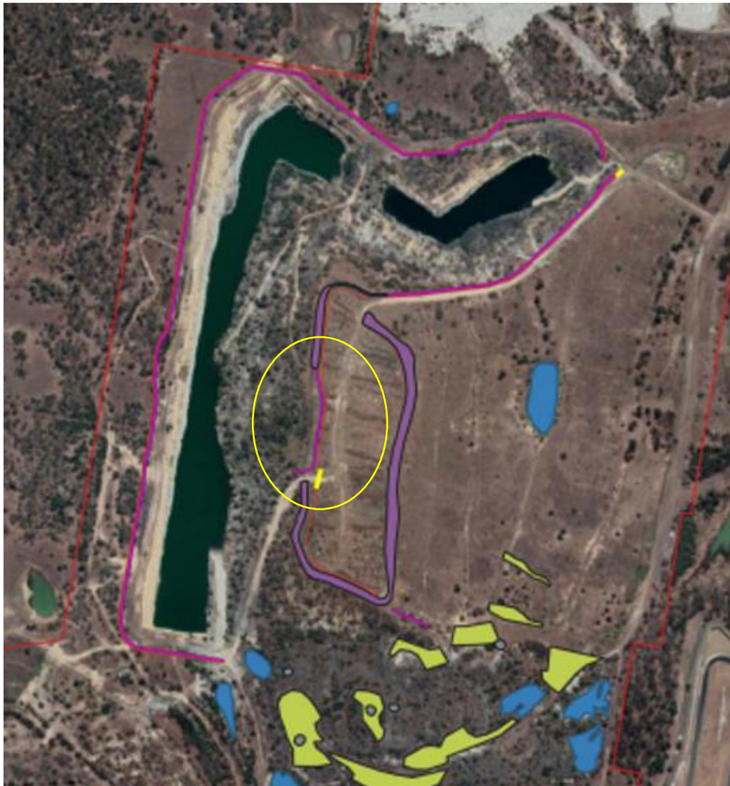
APPENDIX 2 - IMAGE 12: REALIGNMENT OF THE WESTERN BUND WALL
