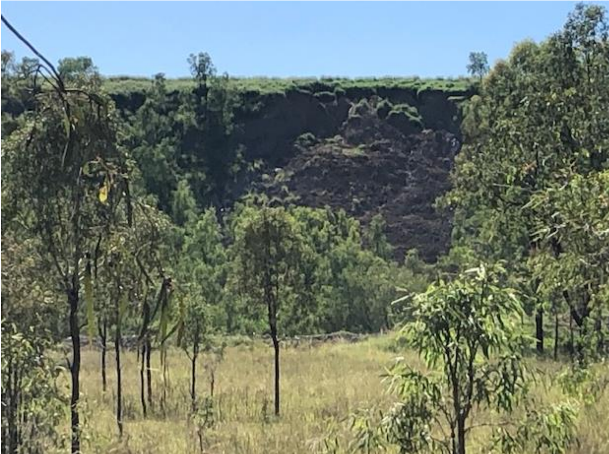
APPENDIX 2 - IMAGE 13: LAND SLIP ON LOW-WALL (15/12/2021)
