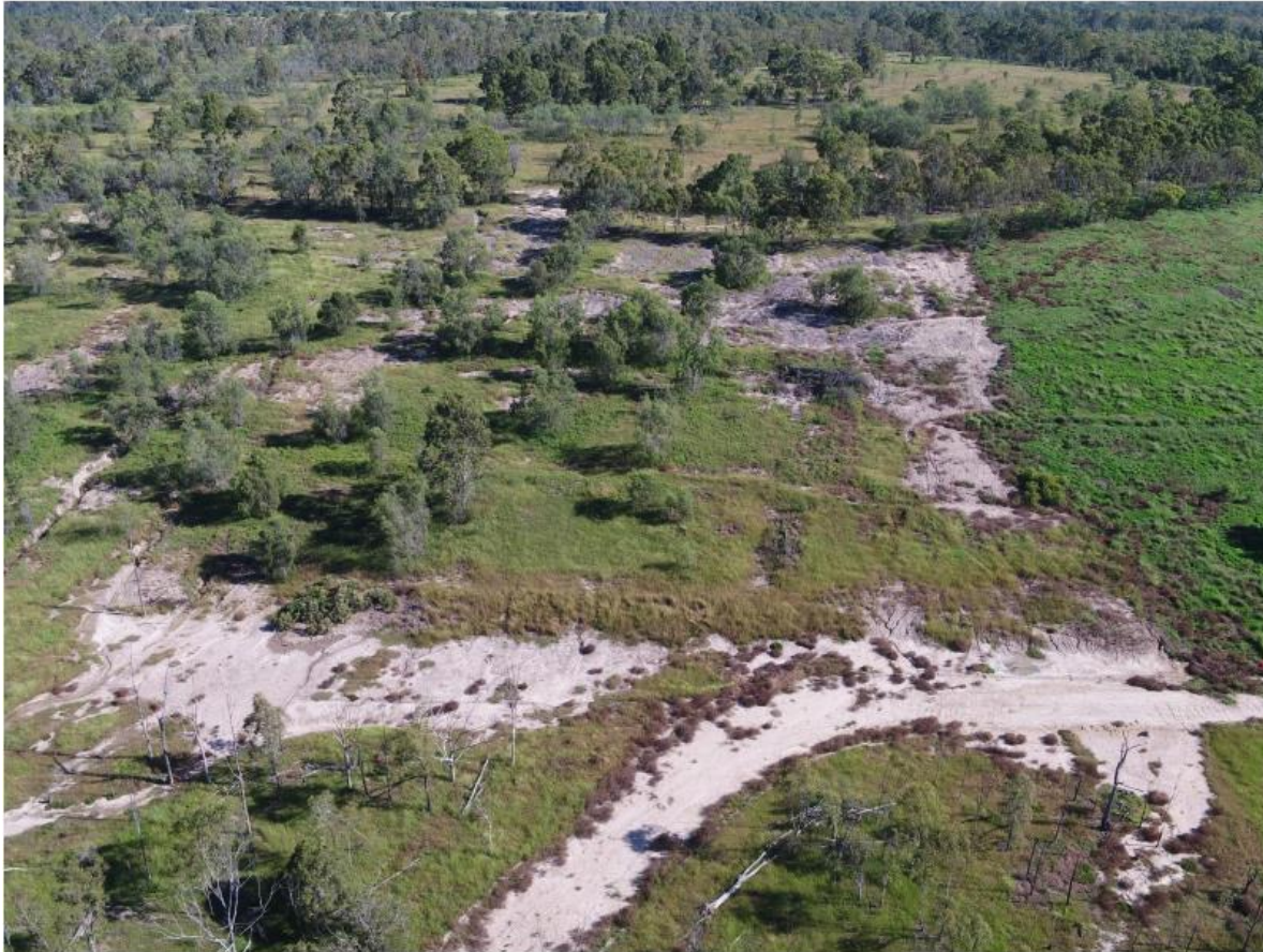
APPENDIX 2 - IMAGE 7: TRANSITION BETWEEN 6 HA AREA OF REPAIRED BATTER SLOPE AND AREA REQUIRING REPAIR
