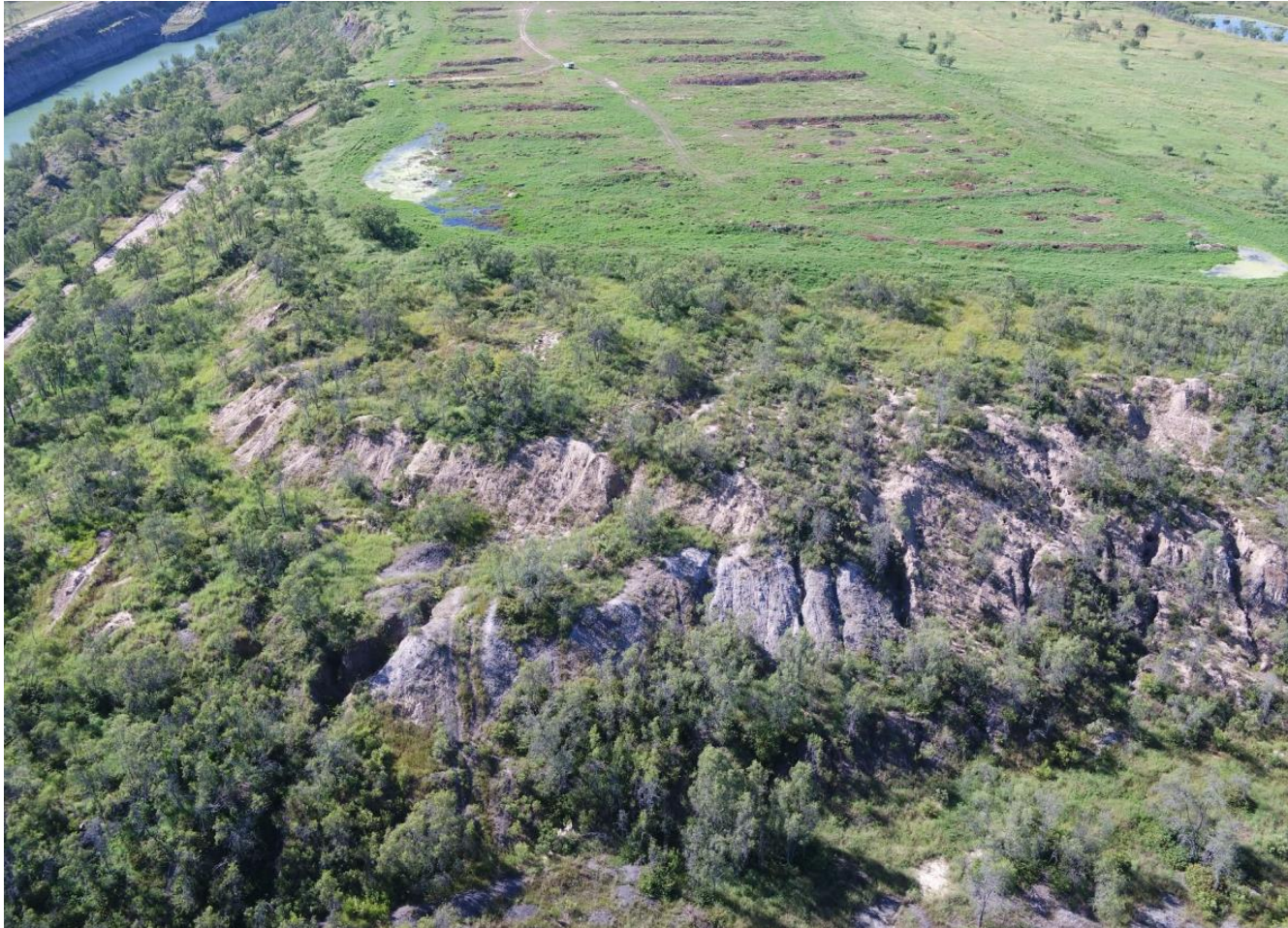
APPENDIX 2 - IMAGE 15: WESTERN SECTION OF IRONBARK SOUTH BATTER SLOPE
