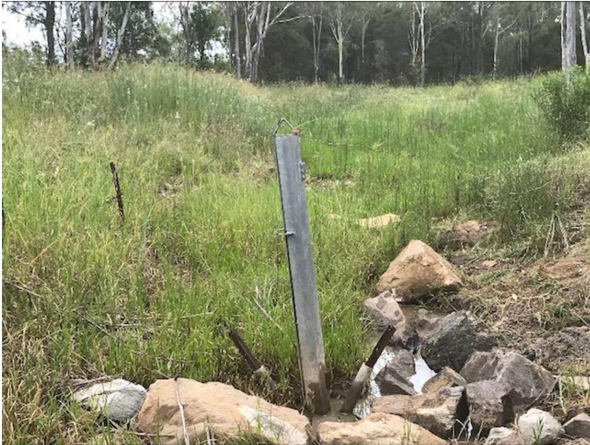
APPENDIX 2 - IMAGE 27: REHABILITATED DRAINAGE CHANNEL AT WATER MONITORING LOCATION EW35 (12/01/2022)
