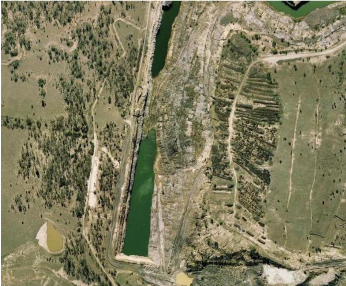
APPENDIX 2 - IMAGE 24: LOW-WALL FAILURE (06/07/2007)
