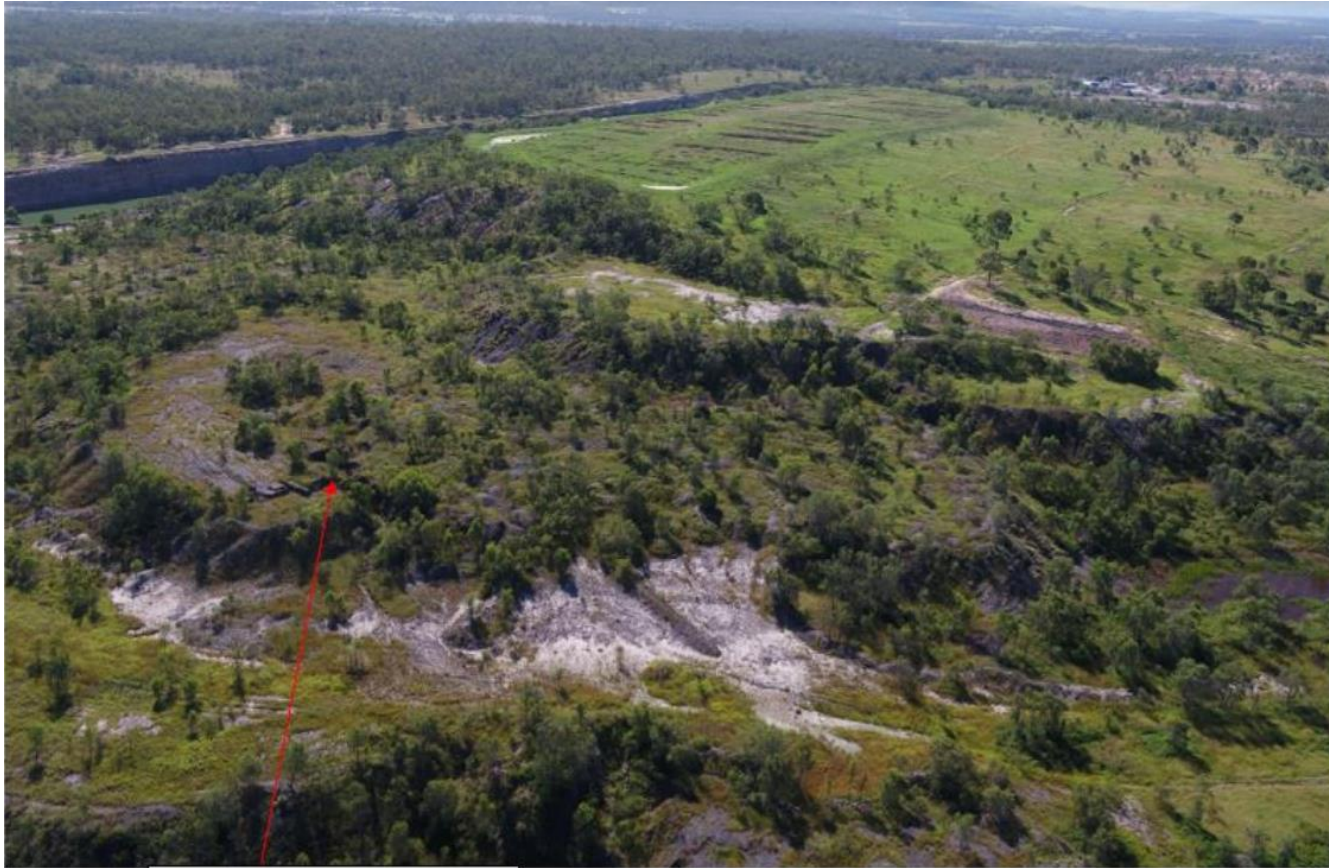
Deep Erosion Requiring Backfilling
