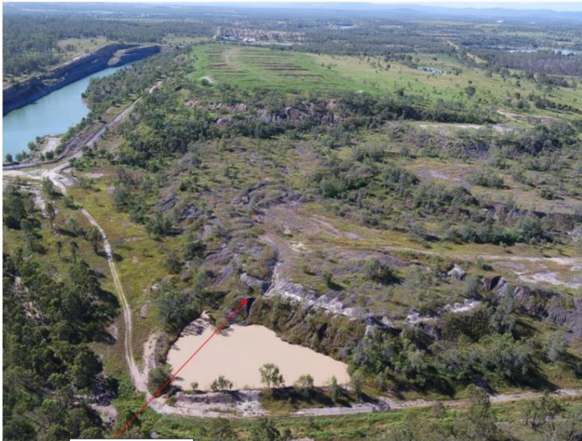
Drain to be stabilised
