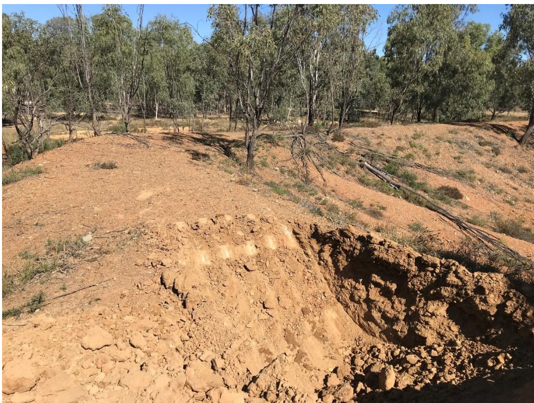
Figure 3.3: Test Pit #5, HL Pond Embankment
