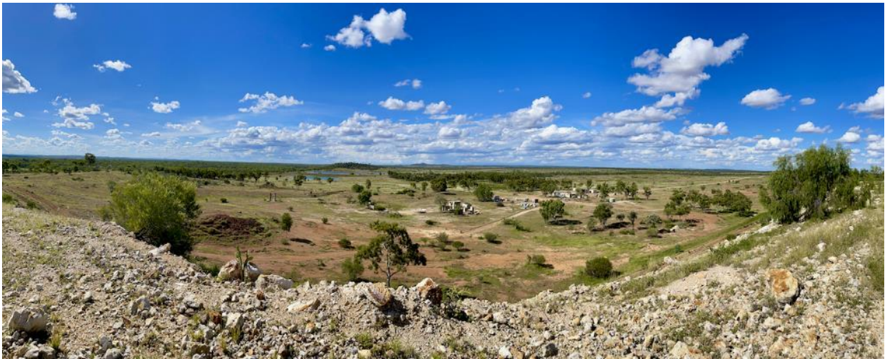
Figure 2 - View north over Yandan project site from top of heap leach pad
