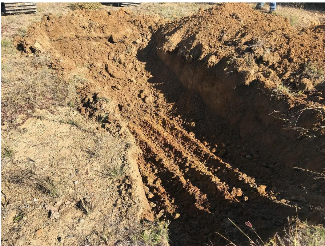
Figure 3.7: Test Pit #18, Topsoil.
