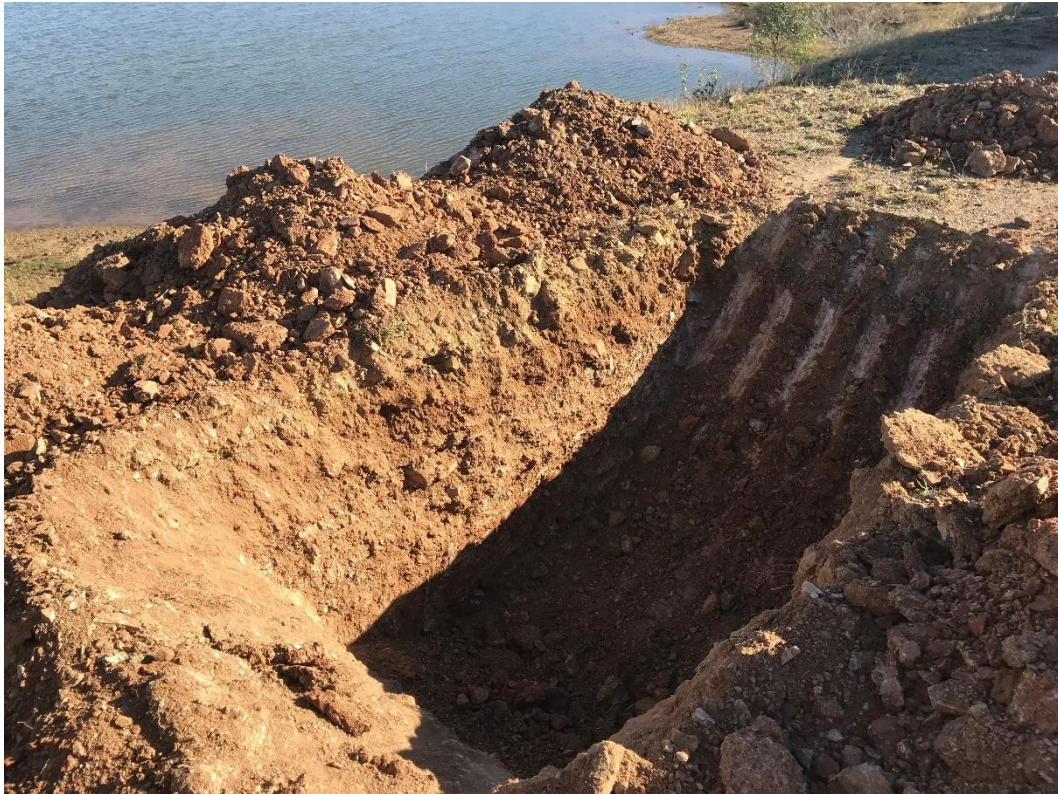
Figure 3.4: Test Pit #7, MWD Embankment (Clay Core)
