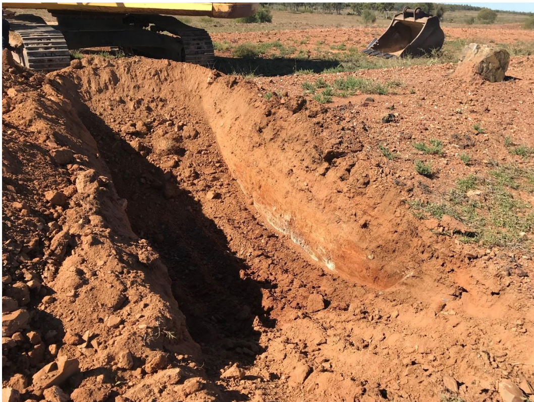
Figure 3.9: Test Pit #15, gravel and topsoil borrow source.
