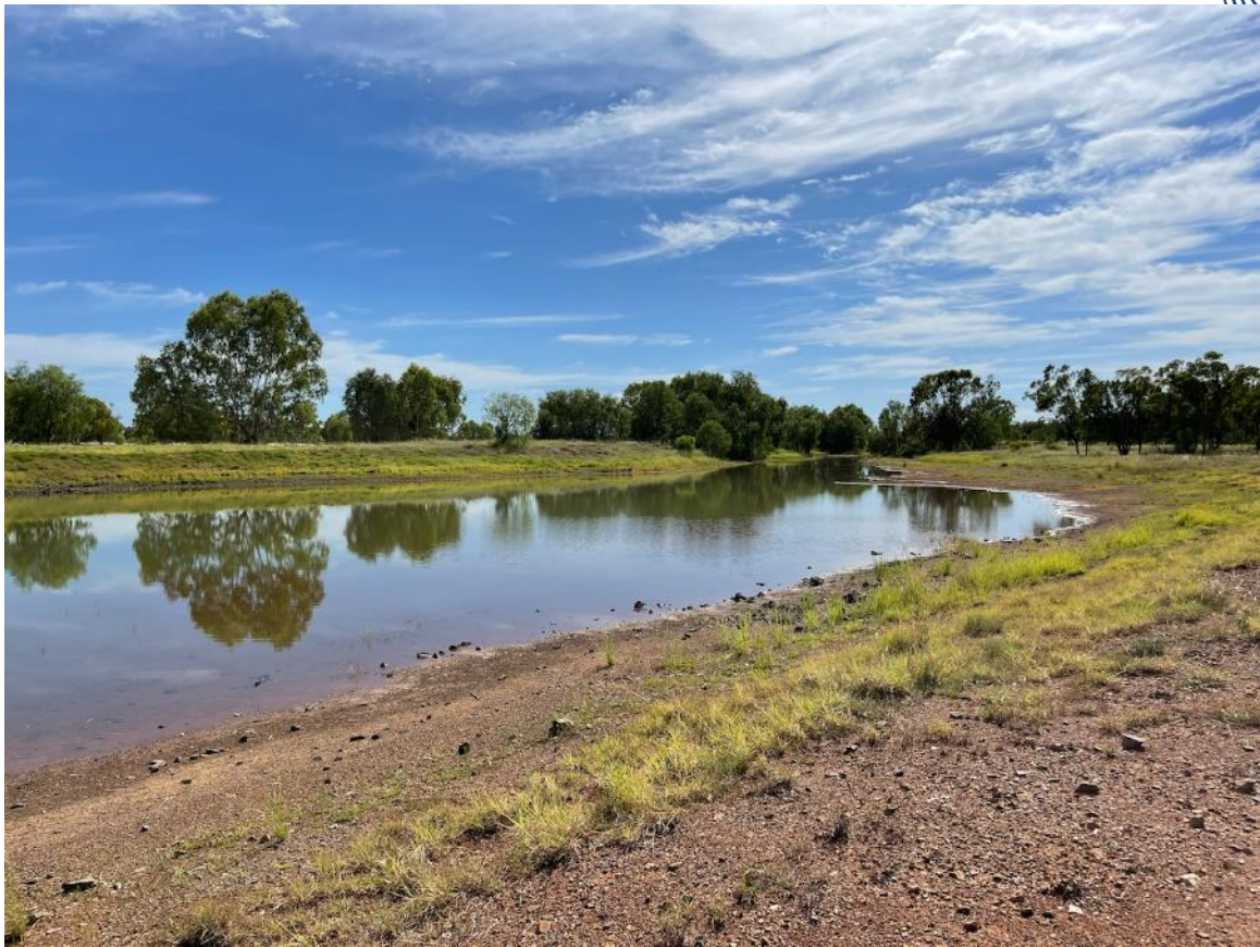
Figure 45 - South borrow pit ponding against embankment (TD Cell B)
