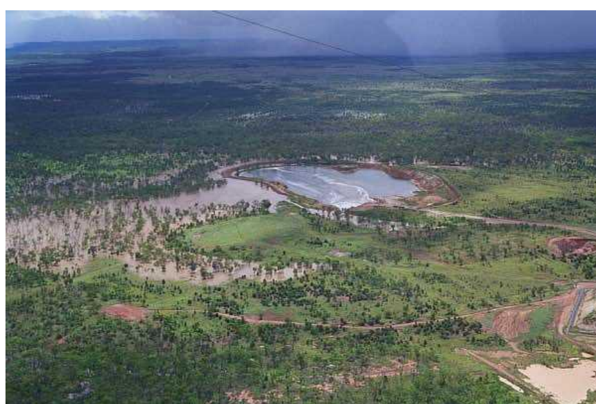
Figure 24 - View of Main pit during flood in 2020
