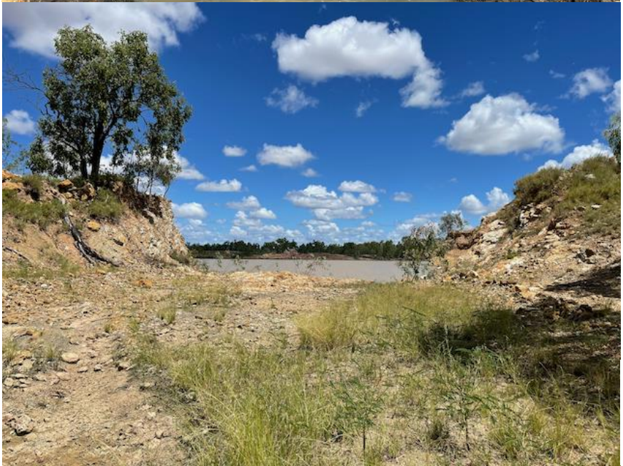
Figure 6 – View of Main Pit northwest spillway
