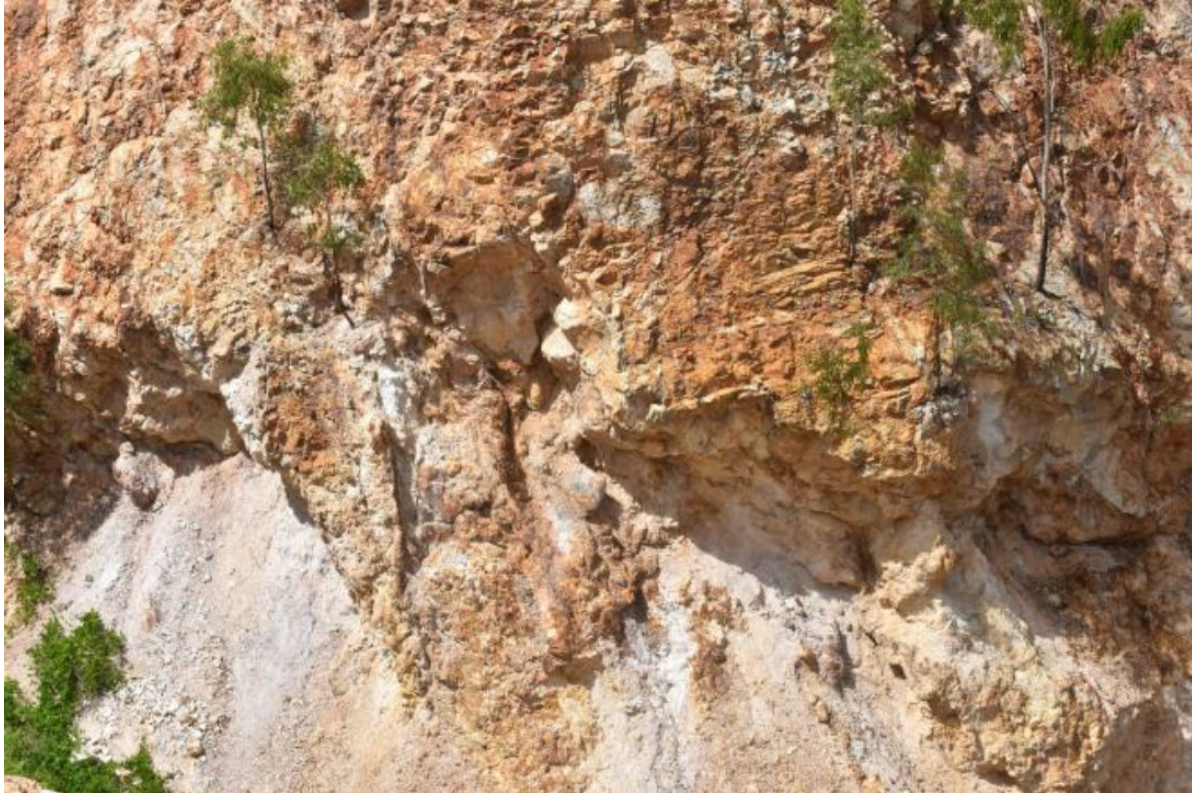
Figure B 9: East Pit Wall Instability - PSM (2021),
