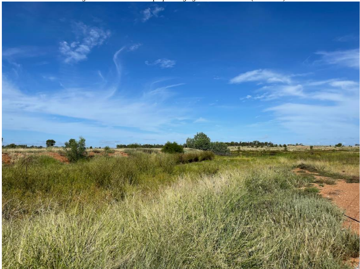
Figure 46 - North borrow pit ponding against embankment (TD5)
