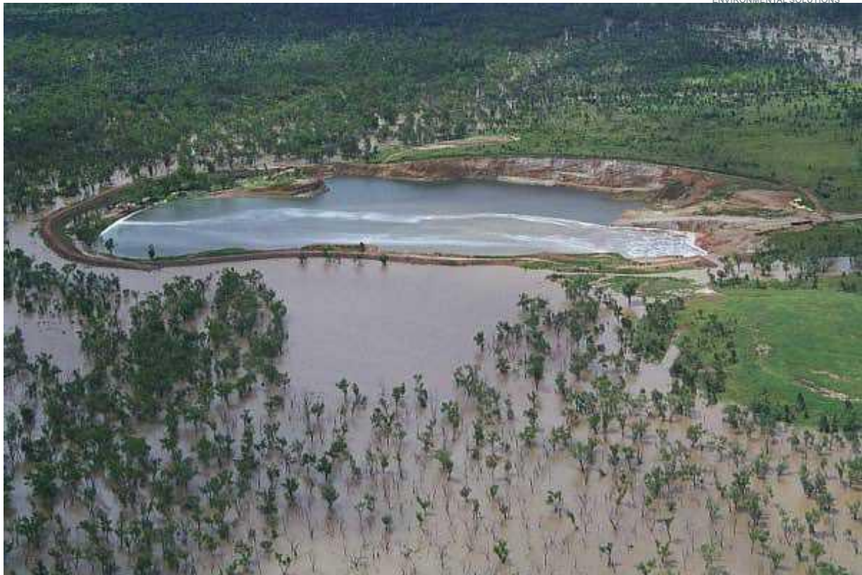
Figure 101: Main Pit inflows during flooding of the Suttor River in February 2020
