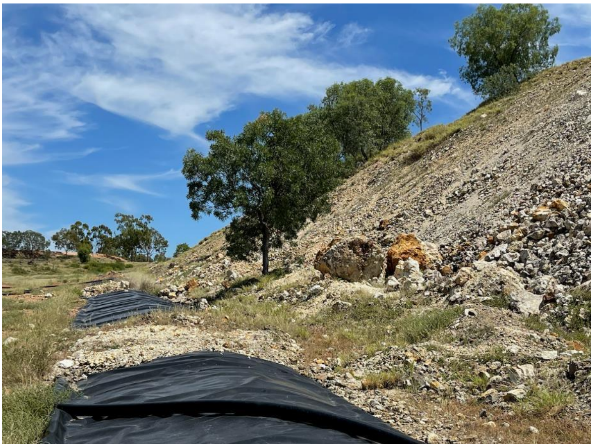
Figure 55 - Views of leach pad drainage with some erosion & minor wall slumping
