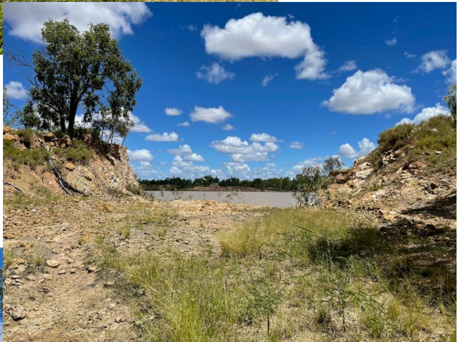
Figure 62 - Views of spillways at south east & north west ends of Main pit
