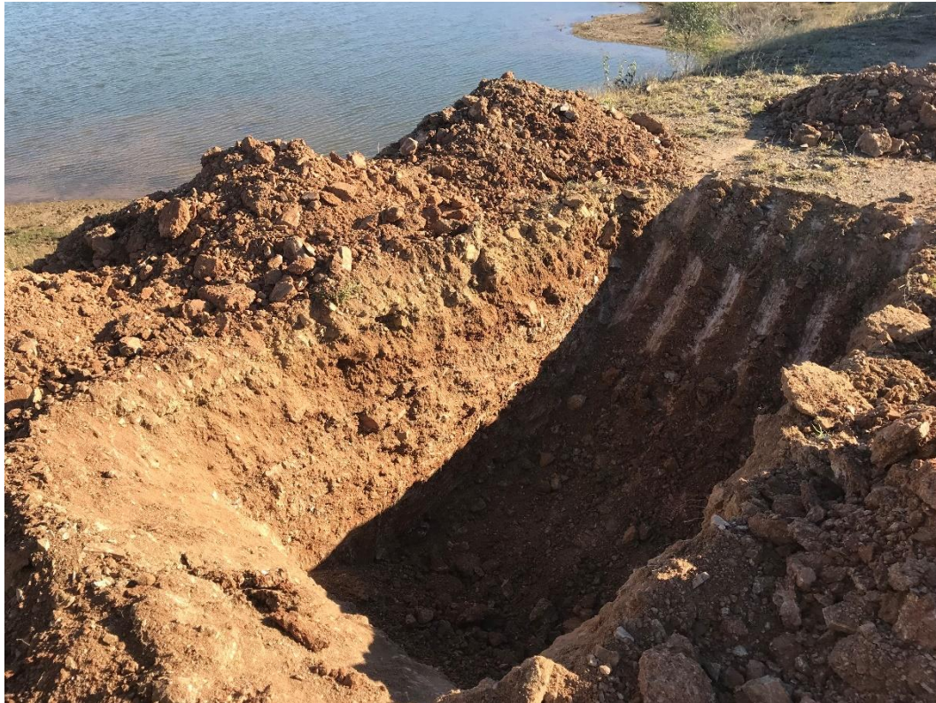
Figure 3.4: Test Pit #7, MWD Embankment (Clay Core)
