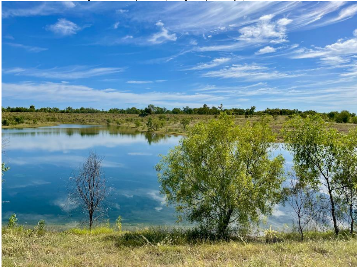
Figure 41 - View from downstream of facility looking at downstream embankment from containment dam
