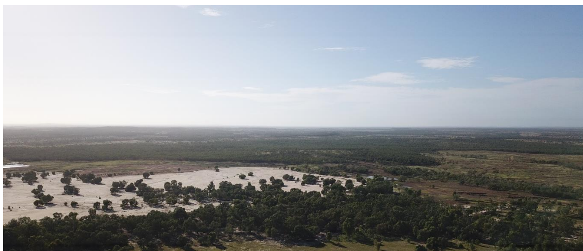
Figure 34: Established vegetation in the drainage channels of Cell B
