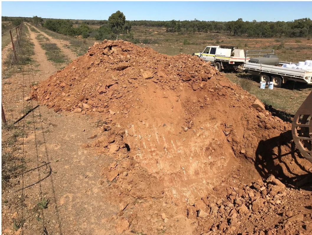
Figure 3.1: Test Pit #13, tailings water dam embankment (clay core)
