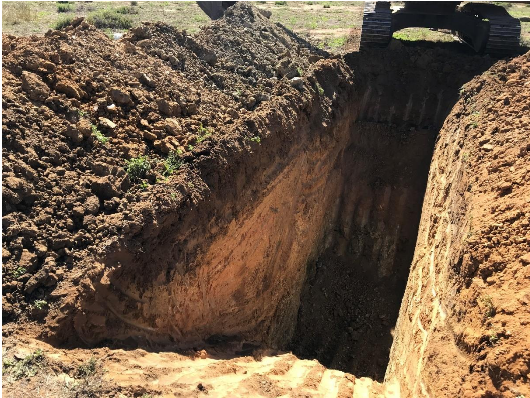
Figure 3.6: Test Pit #11, on-site clay borrow material.
