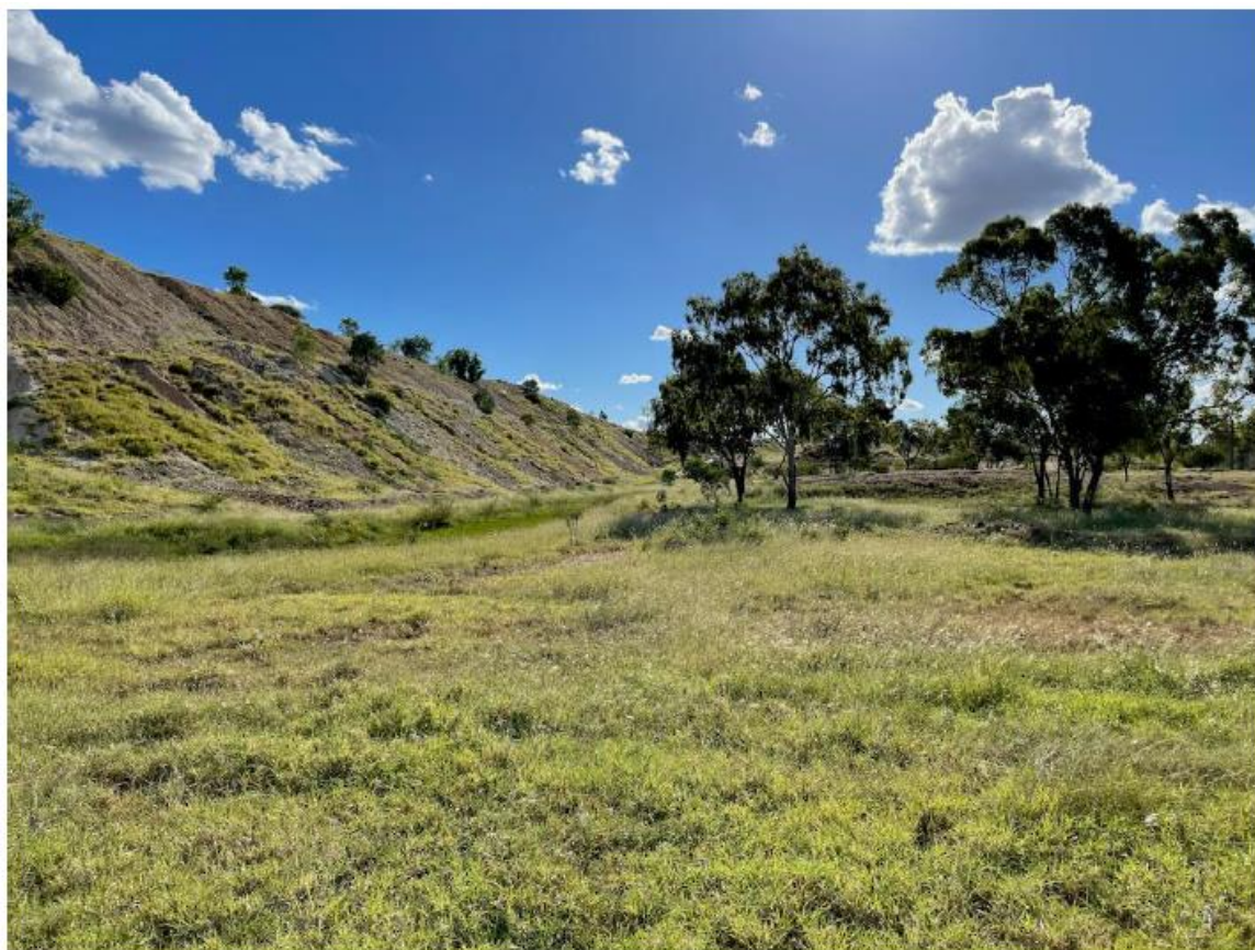
Figure 50: View of Heap Leach Pad (SBE 2022)
