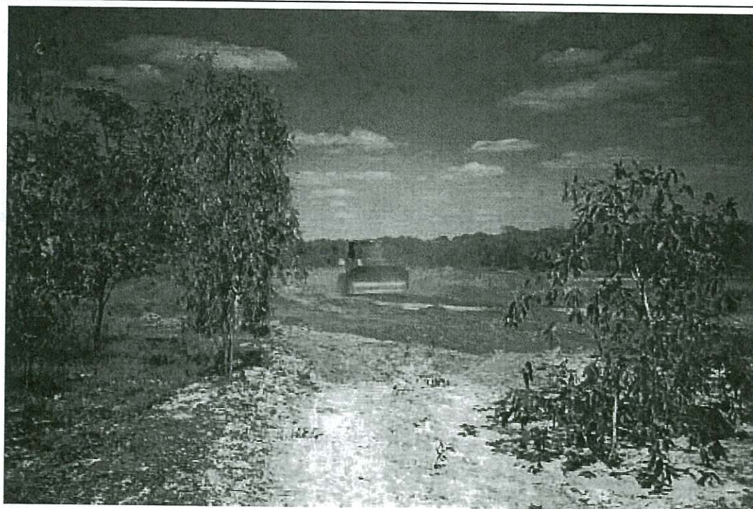
Spreading sand and soil over hardstand area – 9 July 2002
