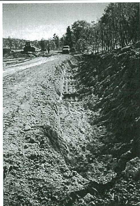
Trench about 52 m long opened up along toe of waste dump with no trace of ARD seepage
