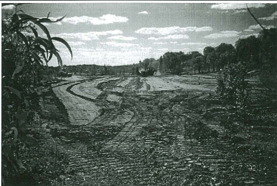
Spreading sand and soil continues over hardstand area – 9 July 2002
