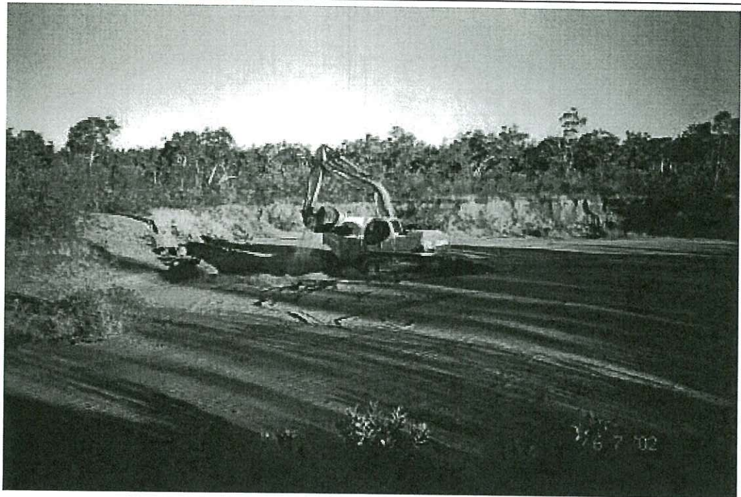
Excavation of sand for backfilling and coverage at Content hardstand area
