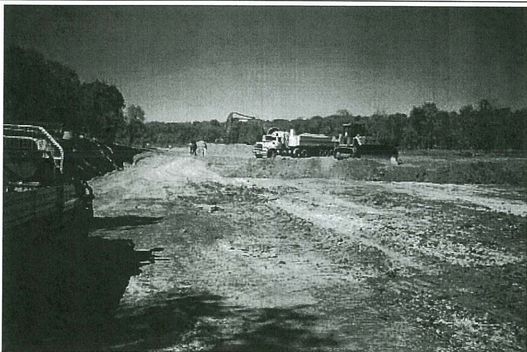
Stripping of surface layer from hardstand area continues – 6 July 2002
