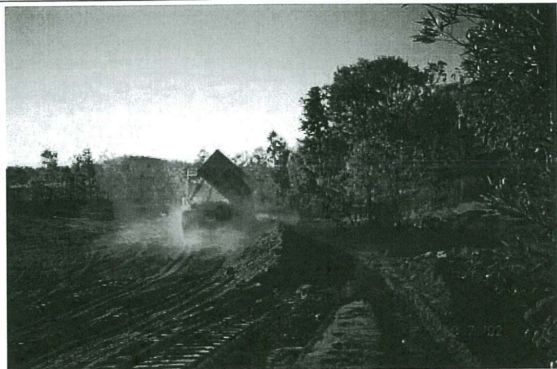
Dumping of sand and soil ready for spreading over hardstand area – 8 July 2002
