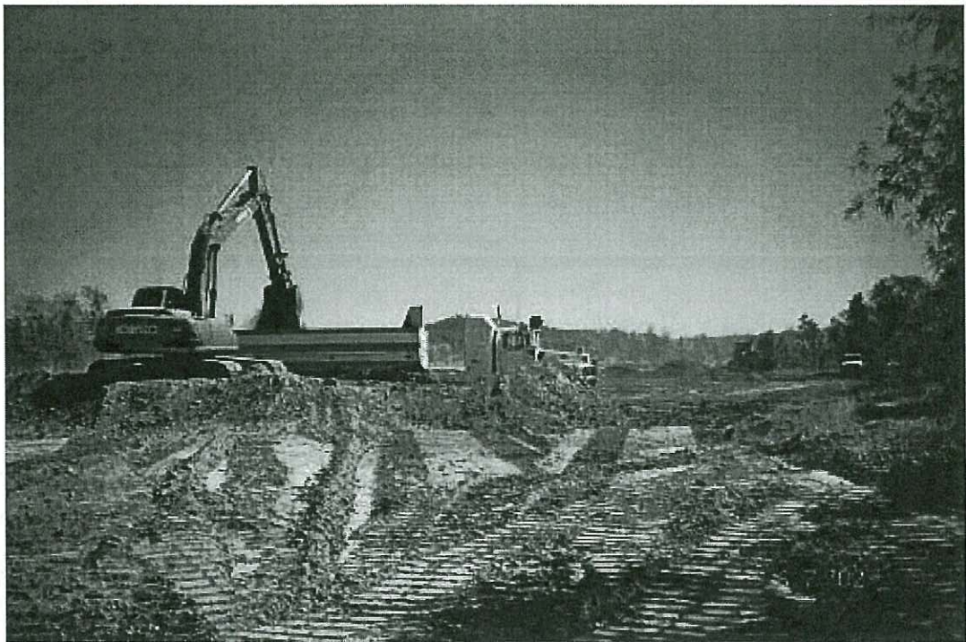
Loading of surface layer material for disposal in Content pit
