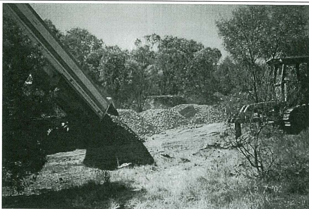
Dumping more screened river rock ready for placing with excavator in drains to Content pit
