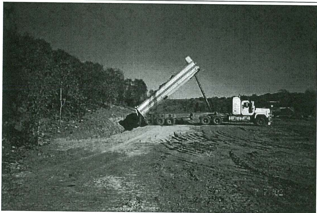
Continuing backfilling of trench
