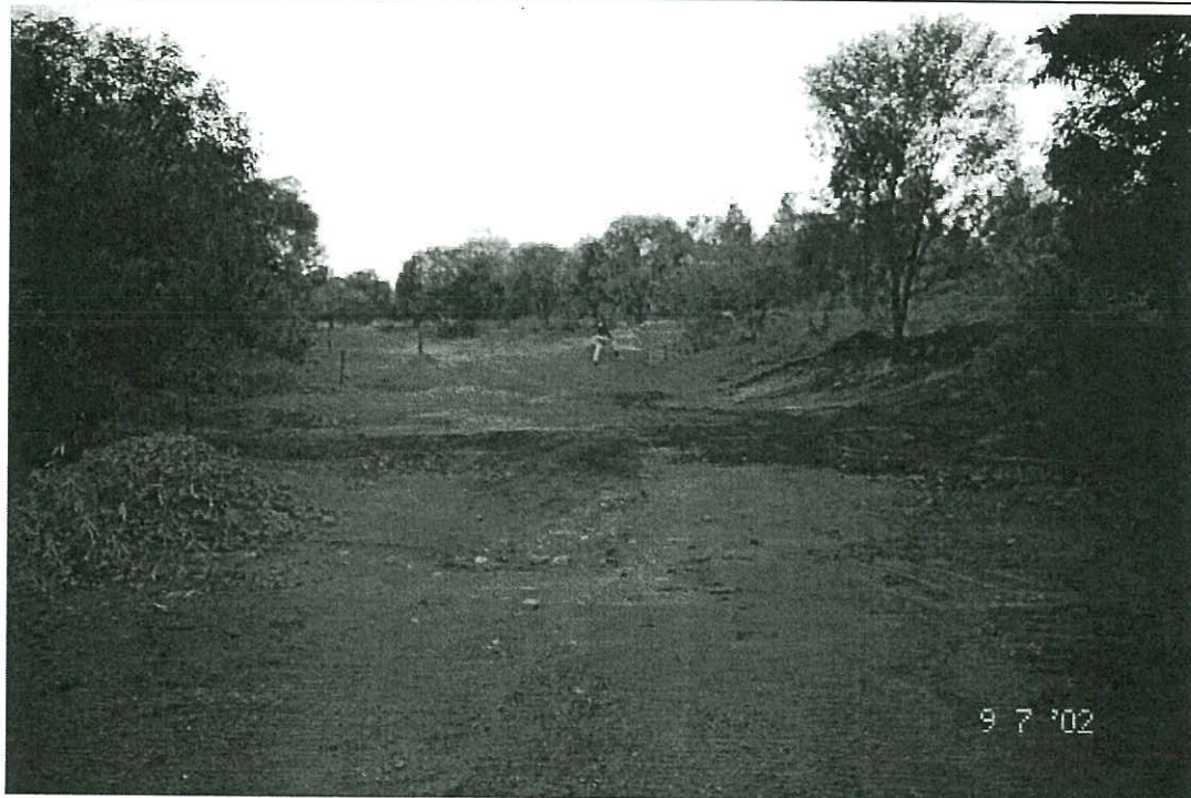
Area between waste dump and Content pit now with 2 cross drains and connecting lateral toe drain, backfilled with screened river rock, compacted and levelled
