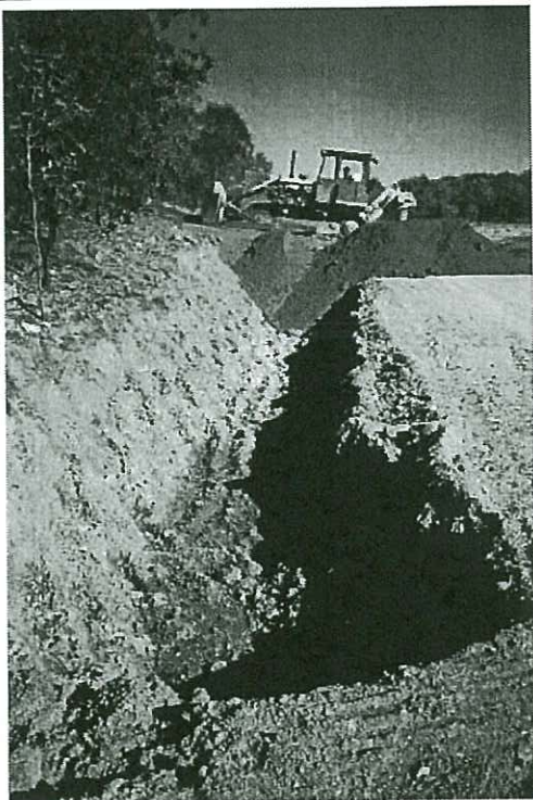
Spreading and compacting trench backfill
