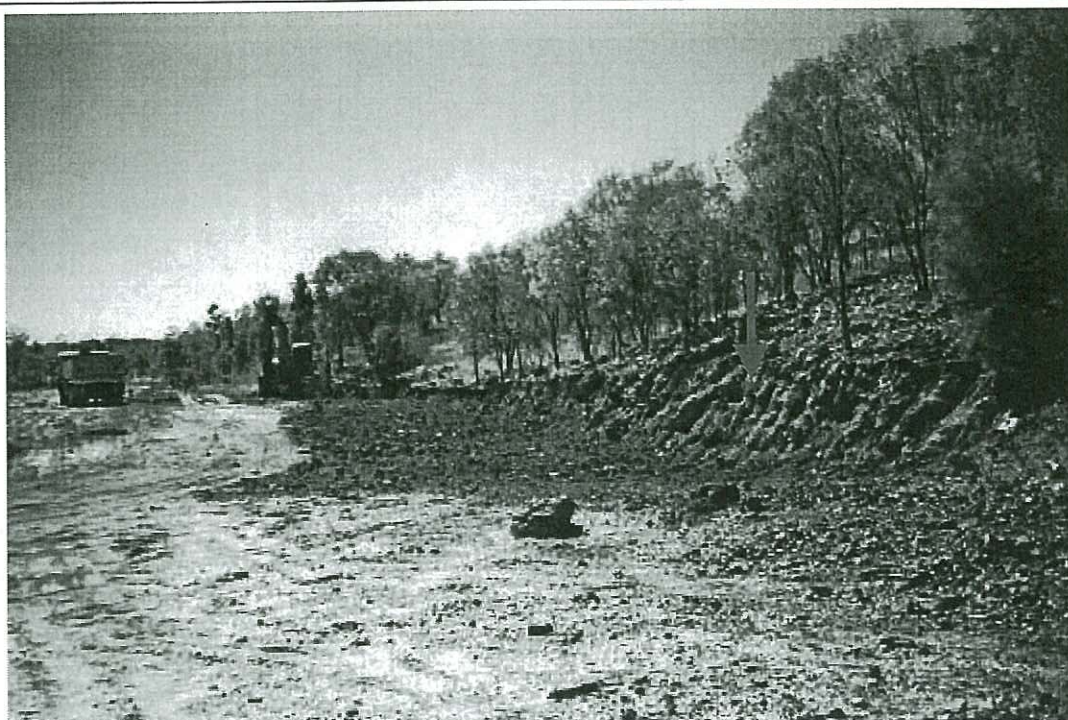
Preliminary cut along toe of waste dump to check for ARD seepage – note red clay layer under loose cover
