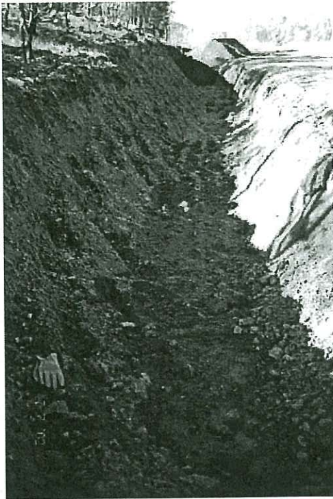
Backfilling trench after finding no indication of ARD – note proximity of high TDS water to surface
