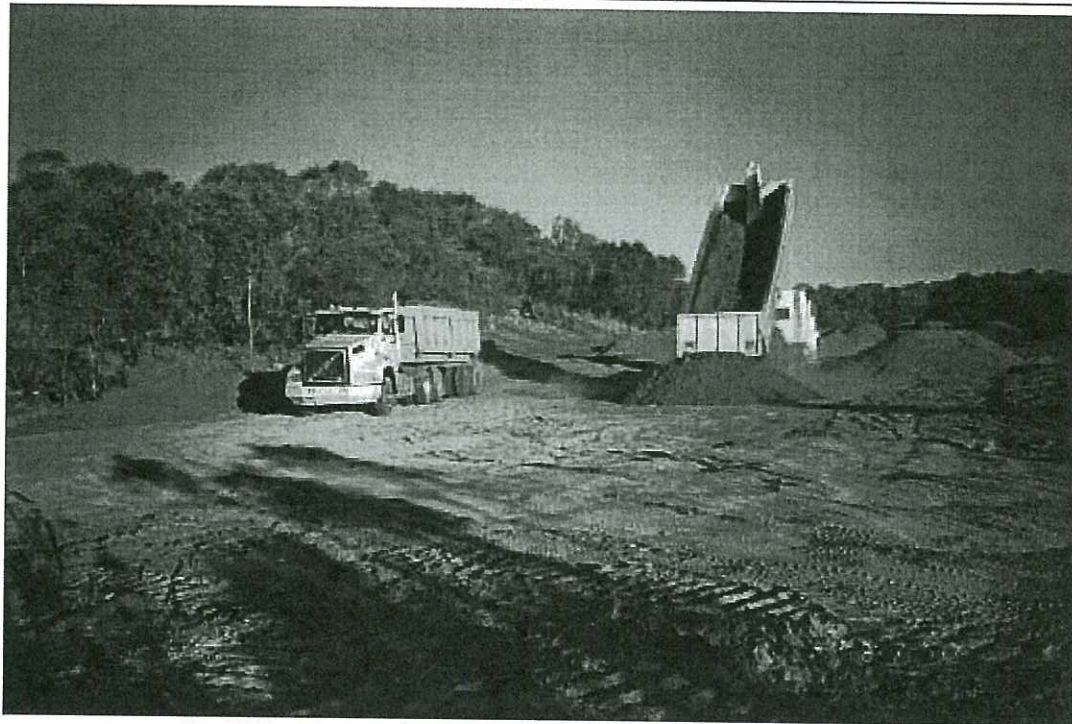
Dumping of sand and soil continues ready for spreading over hardstand area – 8 July 2002
