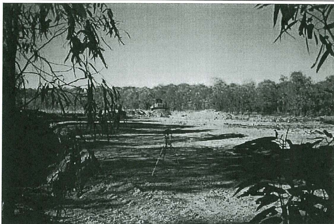
Stripping of surface layer from Content hardstand area – 6 July 2002
