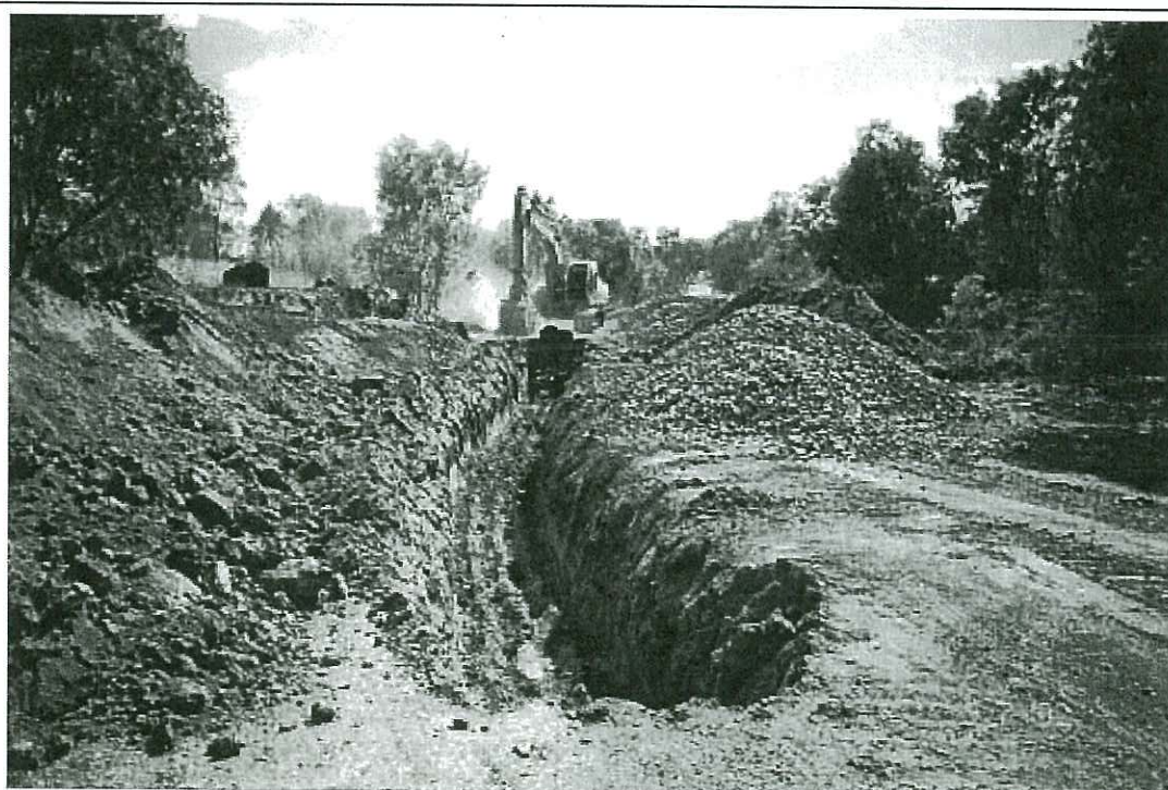
Finishing excavation of lateral waste dump toe drains before backfilling with screened river rock
