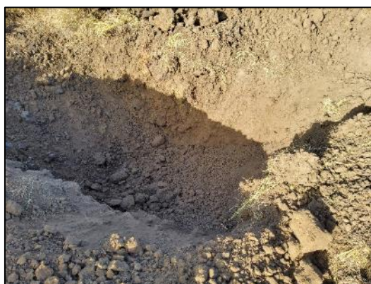
Figure 3: Excavated soil at stockpile 6.
