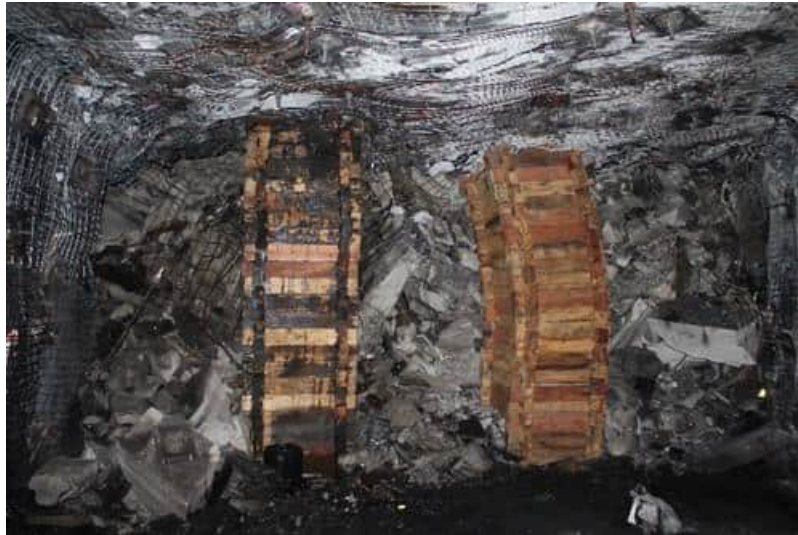
Figure 1 Typical nature of caved material at seam level
