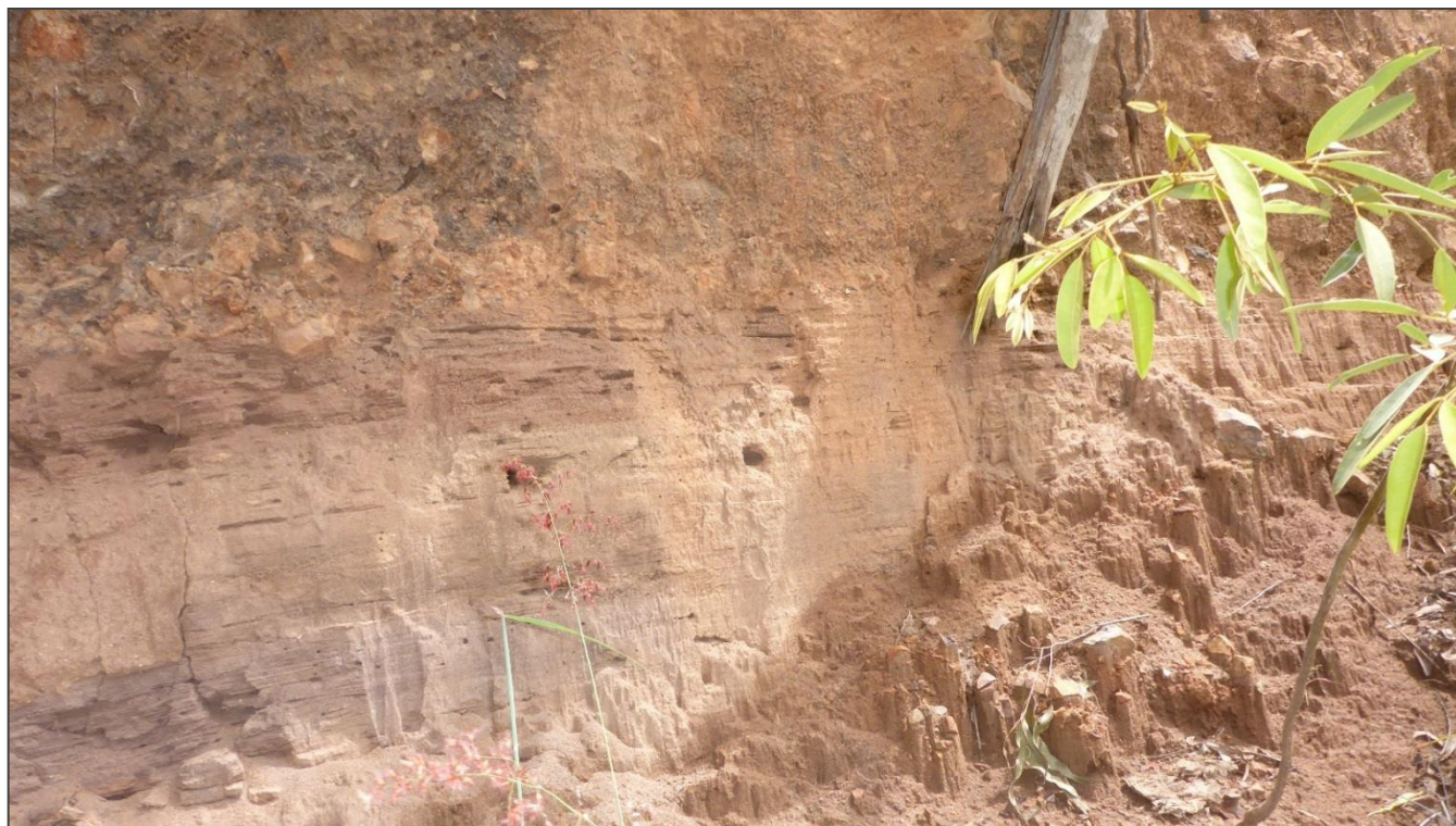
Plate 3-3: Tunnels in bank
