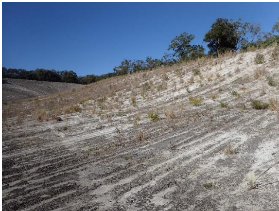
Figure 3-1 North-facing slope of 2019 rehabilitation
