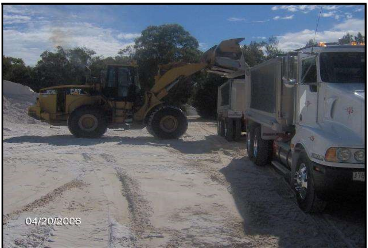
Photo 4. Loading of Haul Truck at the Stockpile Area
