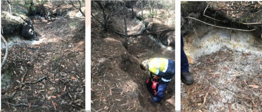
Plate 11 Stabilised erosion features D (left and middle) and H (right)
