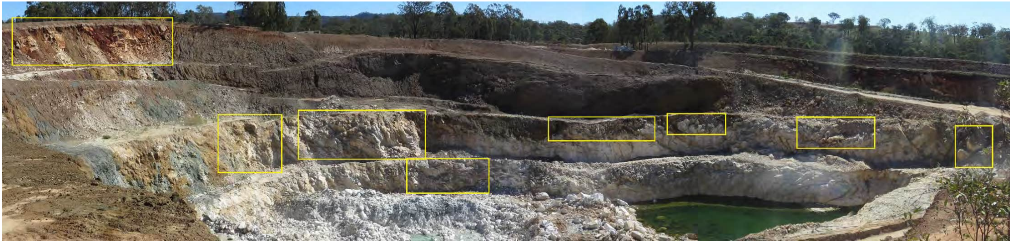
Figure 26. Loss of widths on some berms and scree filled sections of berms, loose rocks on batters and overhanging rocks (highlighted) on the north wall of the Phoenix pit.
