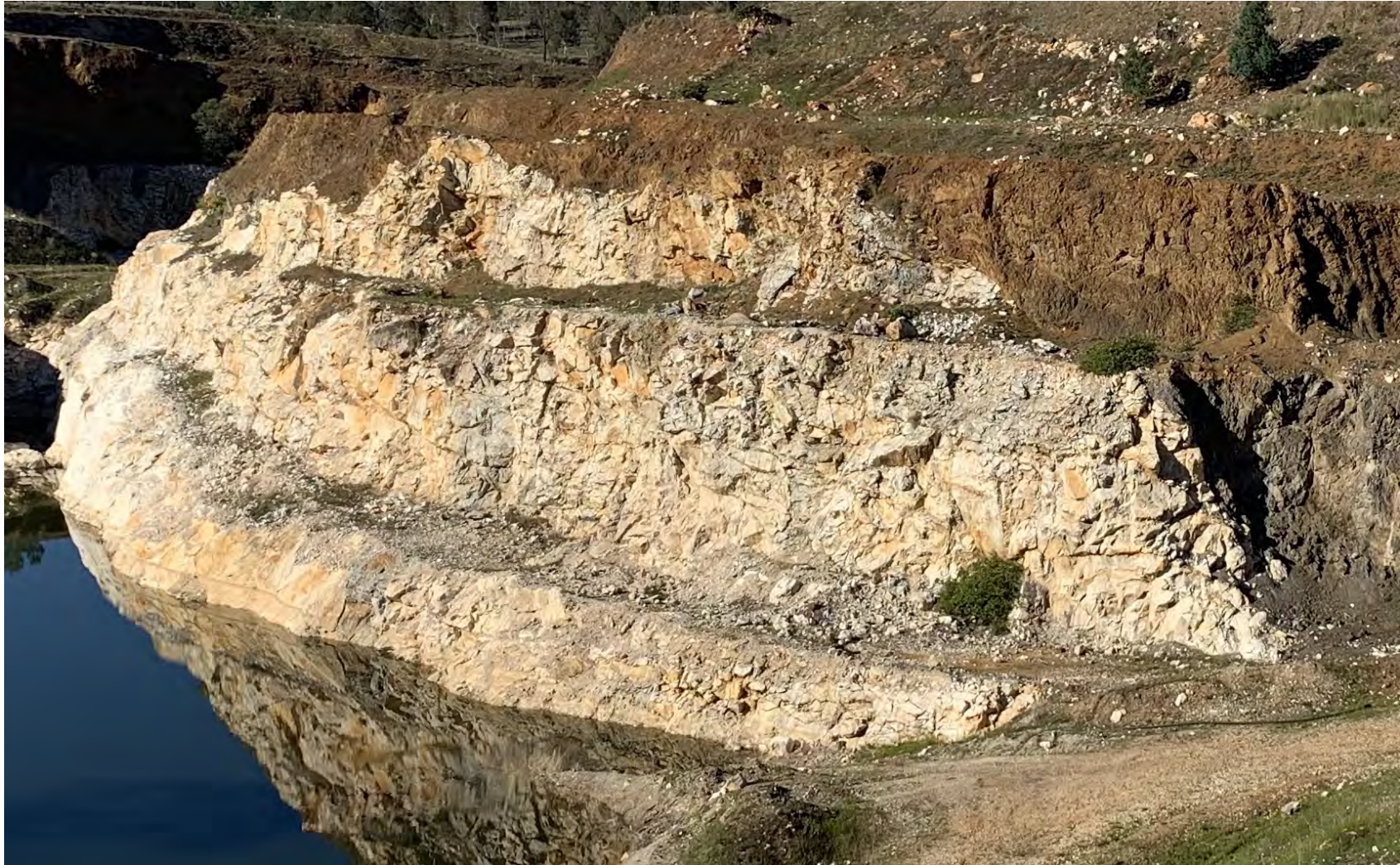
Figure 34. Loss of widths of most sections of the berms and scree filled berms, loose rocks on batters and overhanging rocks on the south wall at the west end of East-West pit. If the adjacent western ramp is to be retained, the height and continuity of the current toe bund are to be increased. Otherwise the ramp will be removed.
