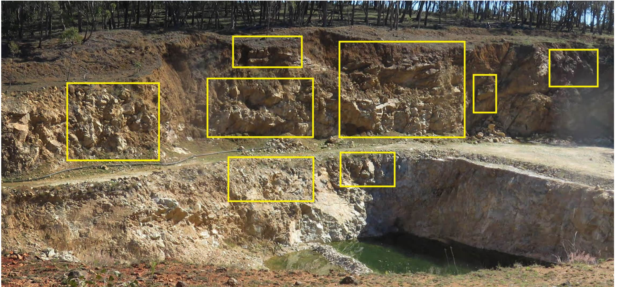
Figure 28. Loose rocks on the batters and overhanging and toppling rocks (highlighted) and scree on the berms on the west wall of the Aspinal pit.
