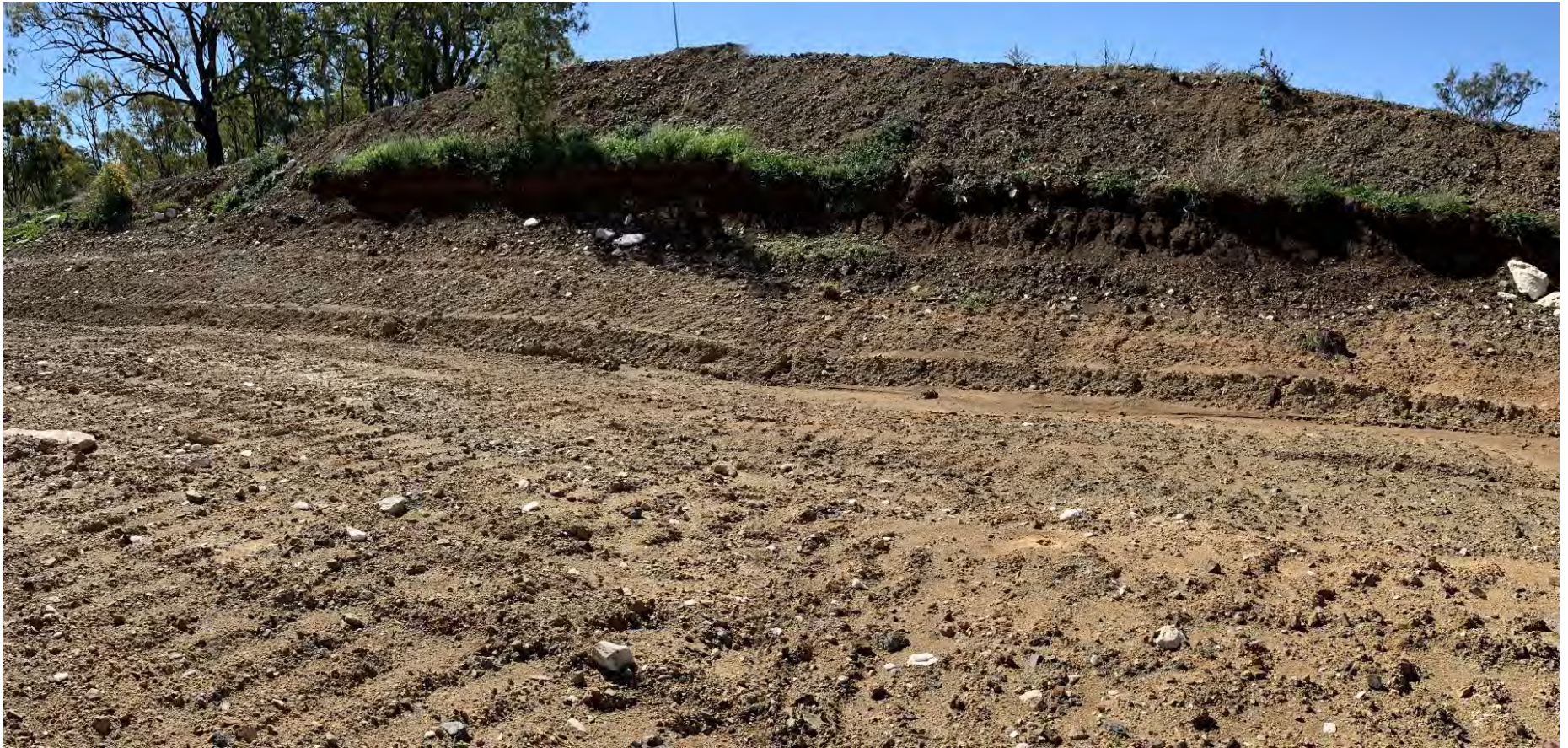
Figure 47. A section of the 3.5-m high bund placed 8-m behind the crest of the east wall of Phoenix pit. Although the offset is less than the 10-m requirement, it is considered acceptable at this location. The haul-road is to be graded to the east, ripped and hydroseeded.
