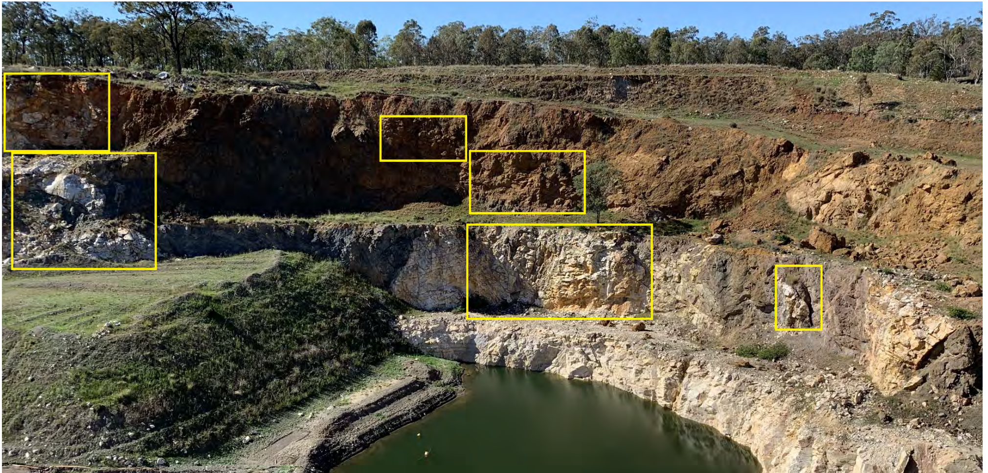
Figure 24. Scree filled berms, loose rocks on batters and overhanging rocks (highlighted) on the northeast wall at the east end of the East-West pit.
