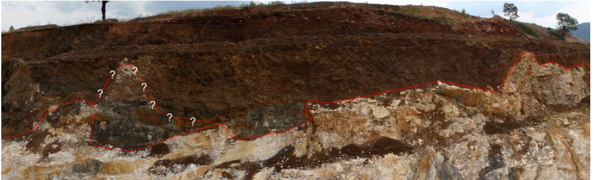
Figure 7. Dissolution has resulted in the upper surface of the limestone being karstified hence irregular. Example is from the south wall at the north end of the East-West pit.
