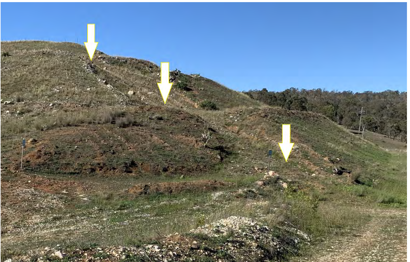
Figure 56. The ramp at the west end of WRD 1 on the south wall of the East-West pit is to be removed by ripping after an abandonment bund has been being installed along the north crest of the dump.
