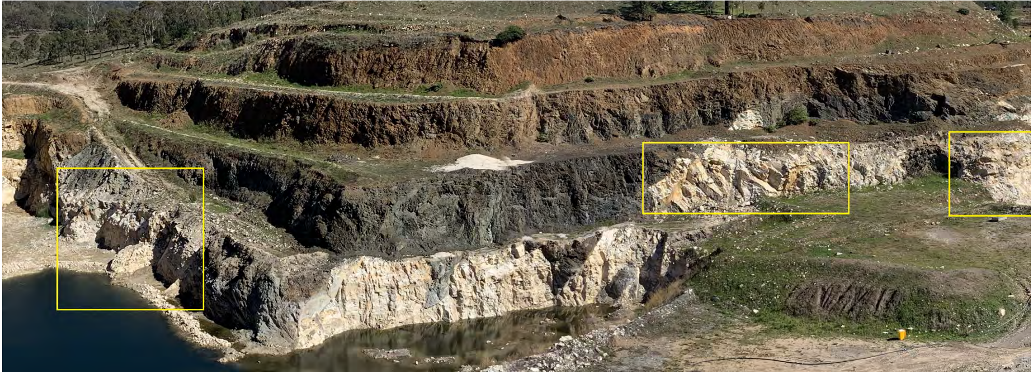
Figure 25. Loss of widths of some sections of some berms, loose rocks on batters (highlighted) on the southwest wall at the east end of the East-West pit.
