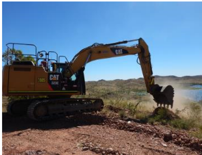
Figure 7-1: Illustration of a test pit excavation
