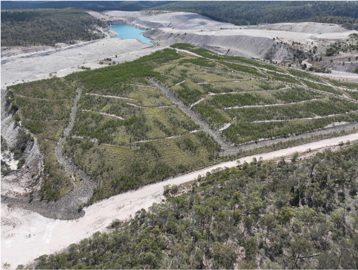
Plate 1: Progressive rehabilitation at the Hut during Yr 2022
