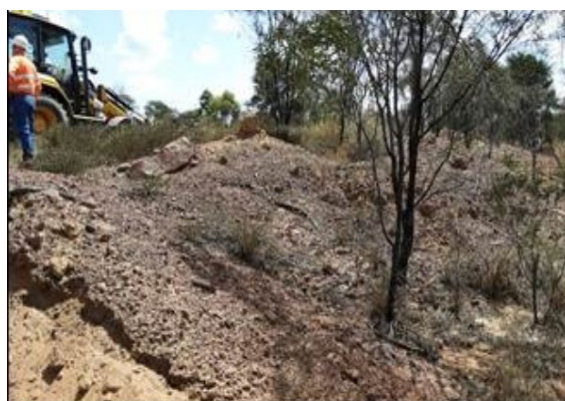
Photograph 14: Vegetation cover on topsoil stockpile 81 is limited and in patches.
