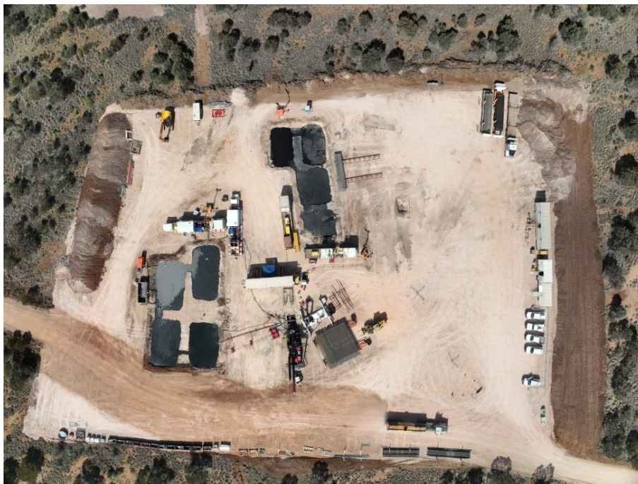
Image 3.2 Example of drill pad arrangement
