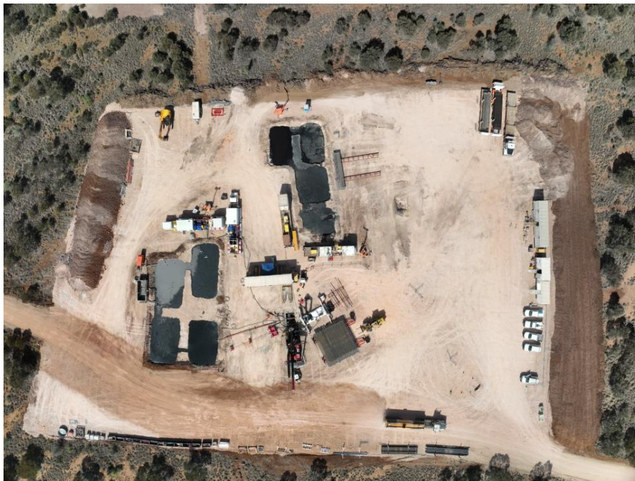
Image 2.2 Example of drill pad arrangement
