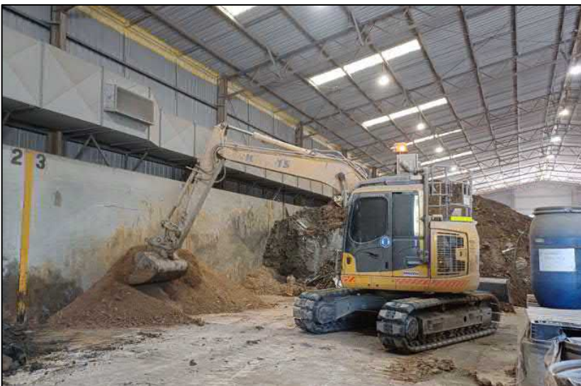
Photograph 7: Homogenisation of soil batches with excavator prior to treatment.
