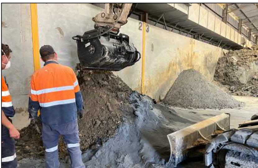
Photograph 10: Application of RemBind 100 to 'batch 3' (Airport soils).
