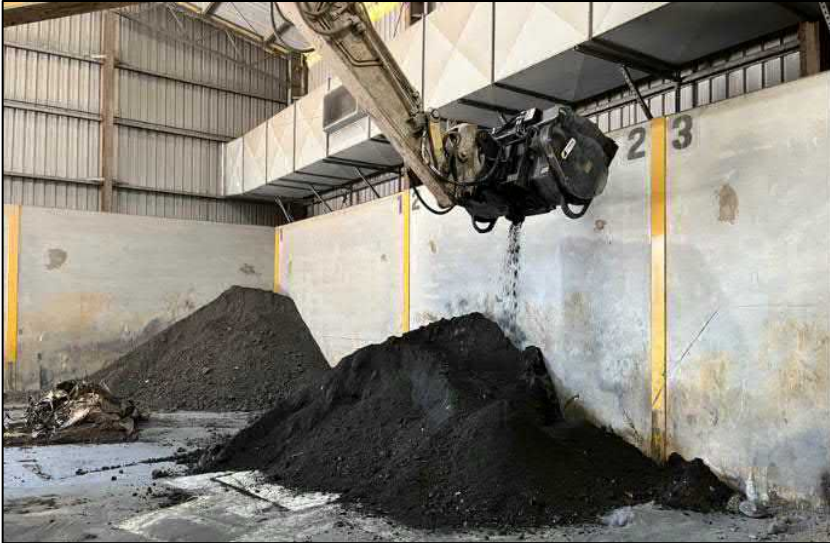
Photograph 11: Application of RemBind 100 to Batch 3' Airport soils.
