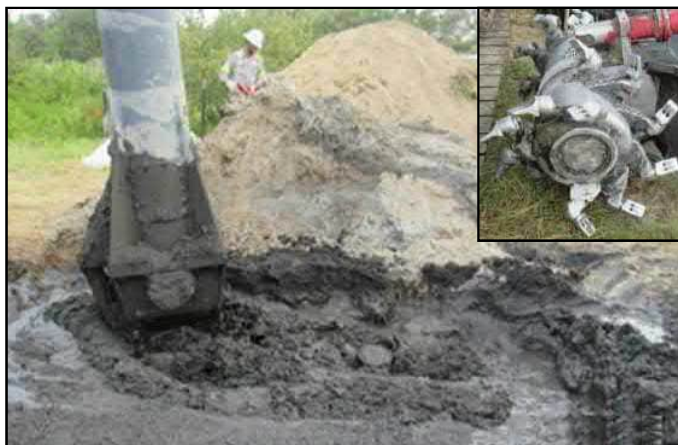
Adding RemBind and Portland cement to immobilise PFAS contaminants at a US field site
